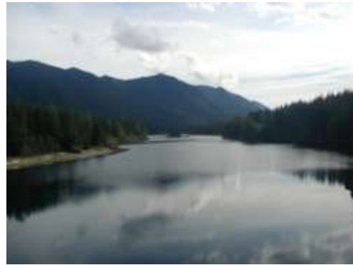
Masonry Pool Reservoir on October 2, 2011
