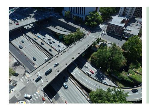
"Most of I-5 coming into and through downtown is on bridges and elevated structures that, without seismic retrofits, will not likely be useable after a strong earthquake. Damage to them would impair emergency services and economic activity for months, if not years."
