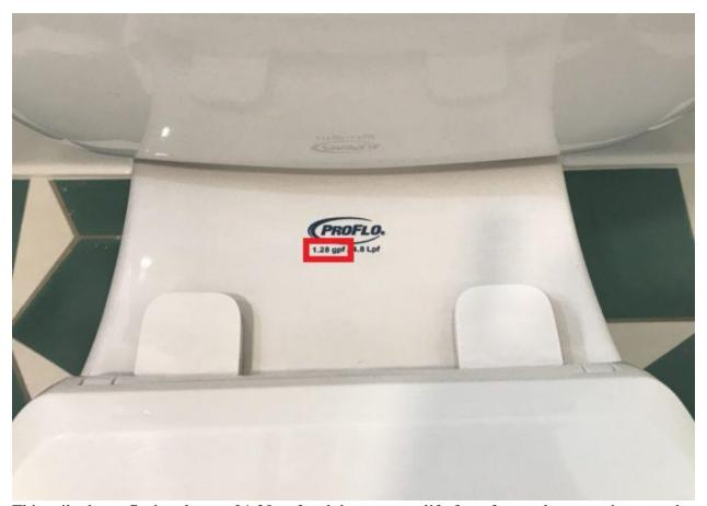
This toilet has a flush volume of 1.28 gpf and does not qualify for a free replacement because the toilet is already considered to be one that saves water.
