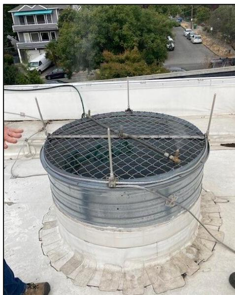
**Figure 5: EF2 Stack Exhaust with Spray Nozzles**
