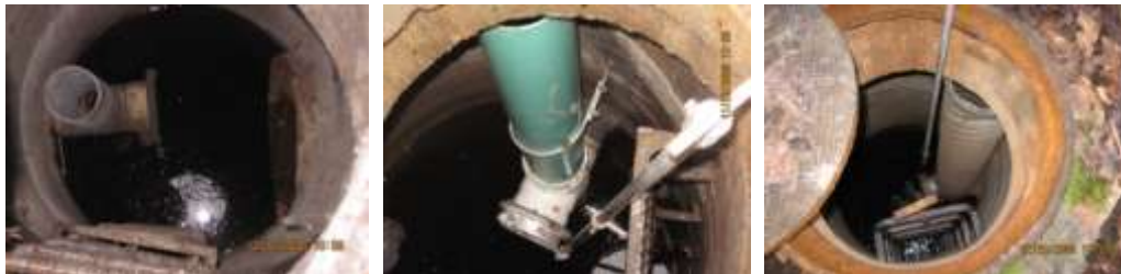
Detention System (Flow Control Structure)
