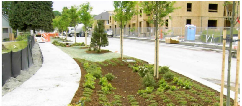
Figure 3. A newly planted natural drainage system
