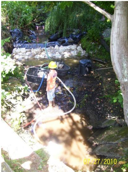
**Tip:** For any stream bypass longer than about 50 ft, consider including intermediate pumping (and possibly discharge) locations.
