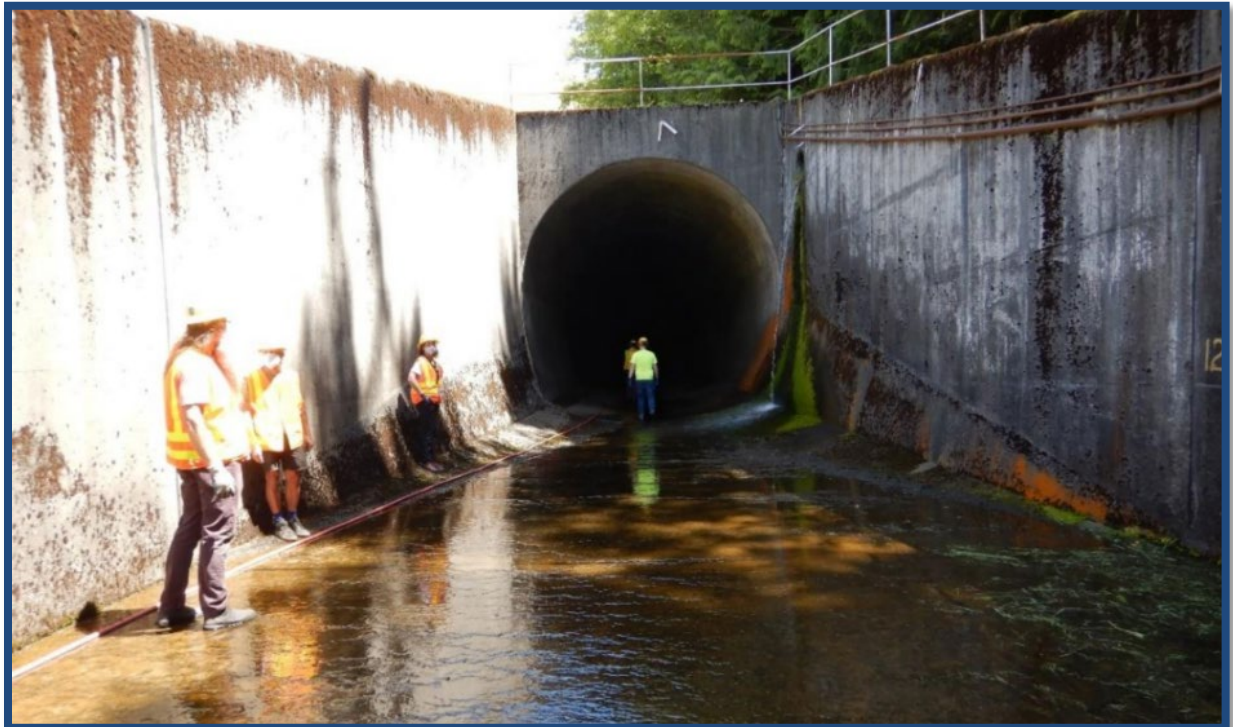
Figure 3.2 – Recent FERC inspection of spillway outlet tunnel.
