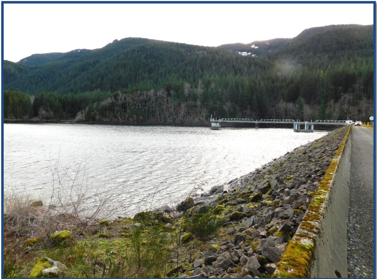
Figure 2.3 – The rock-lined upstream slope of the Tolt Dam embankment and South Fork Tolt Reservoir.
