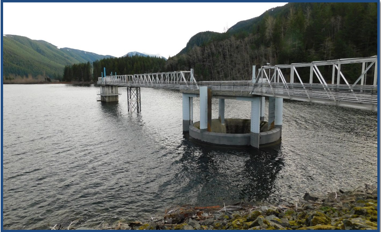
Figure 2.5 – The morning glory spillway inlet (foreground, right side) viewed from the crest of the dam. A bridge leads from the spillway inlet to the top of the outlet works control tower (left side).
