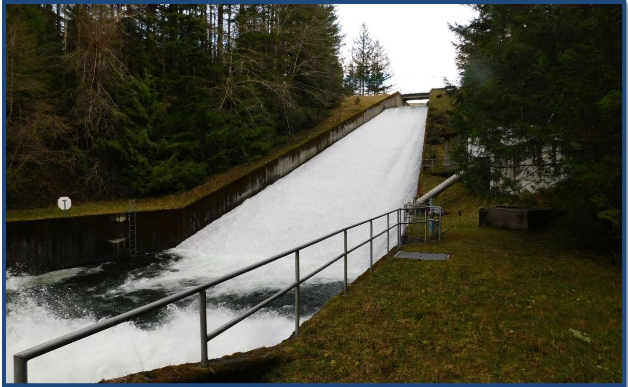
Figure 2.8 – Discharge chute at the downstream end of the spillway outlet channel.
