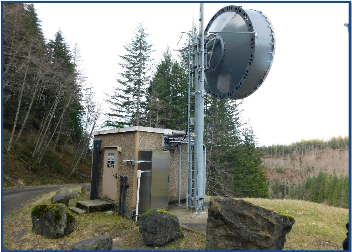
Figure 2.19 – The Tolt Dam microwave radio transmission facility provides redundant communications with the City of Seattle Operations Control Center.
