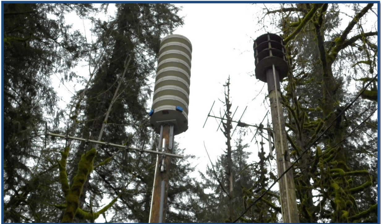
Figure 2.20 – Pole-mounted sirens located on Tolt River Road (old siren shown on right, new siren shown on left).
