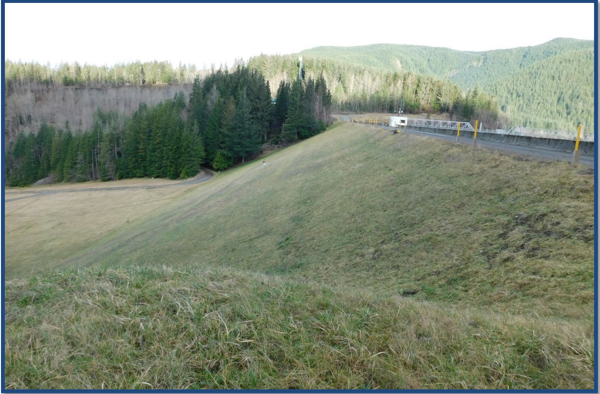
Figure 2.4 - The downstream slope of the Tolt Dam embankment.
