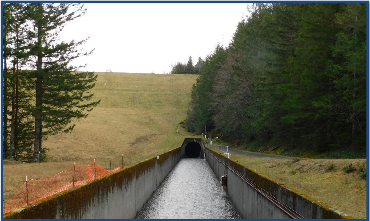
Figure 2.7 – The downstream slope of the Tolt Dam embankment and outlet channel of the combined morning glory spillway and outlet works tunnel.
