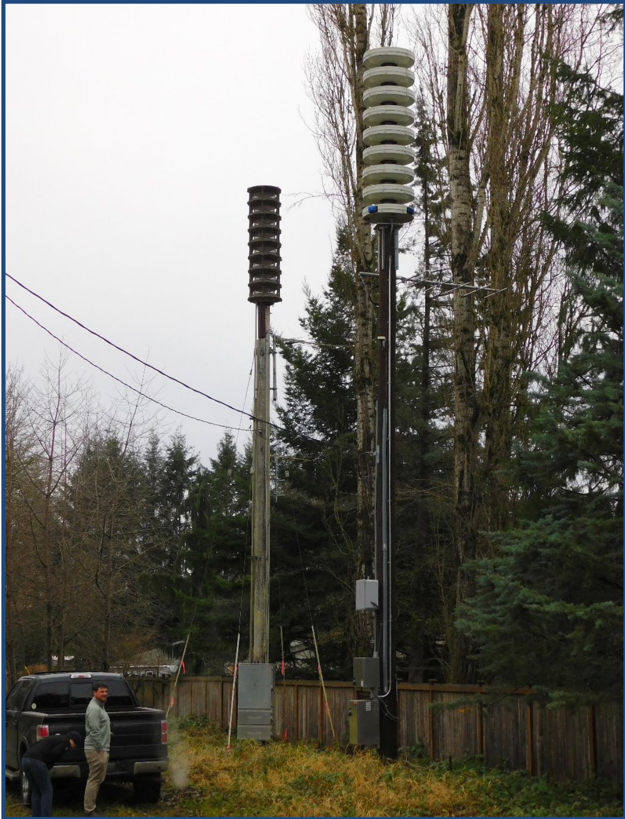
Figure 2.21 – Pole-mounted sirens located in downtown Carnation (old siren shown on left, new siren shown on right).
