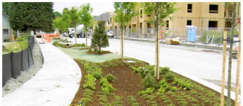
Figure 3. A newly planted natural drainage system
