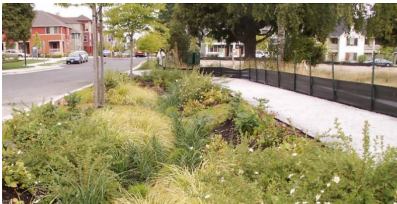
A completed natural drainage system.
