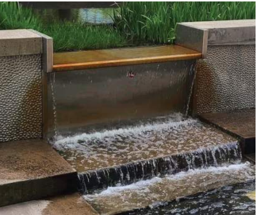
3 Stepped spillway enhanced with material and texture choices
