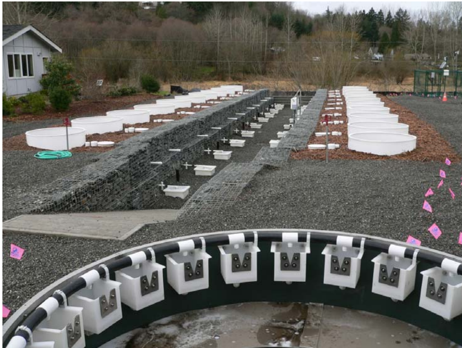
Figure 4.3.1c. Photograph of Cistern and Mesocosm Tanks
