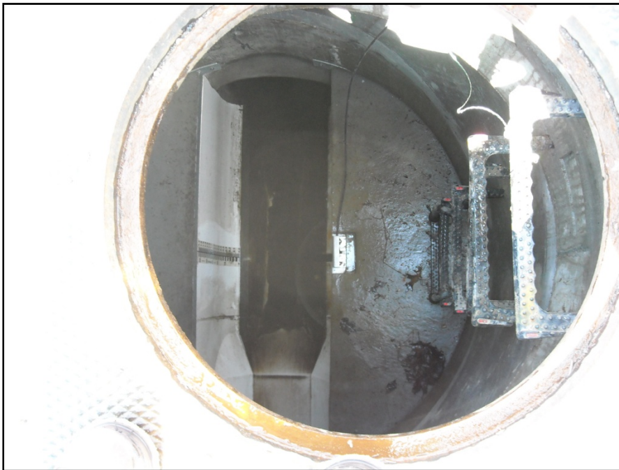
Figure 2.2.2.1b. Photograph of R1 Palmer-Bowlus Flume
