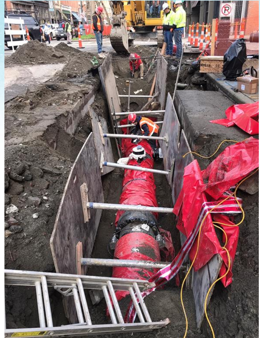
Earthquake resistant pipe installation in Pioneer Square
