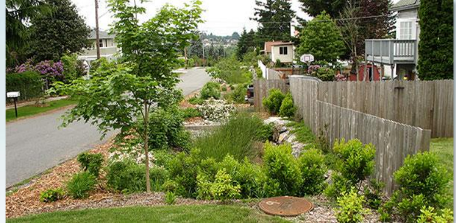
Example of a natural drainage system project a few years after installation
