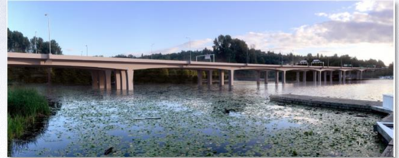
Photo: New bridge
