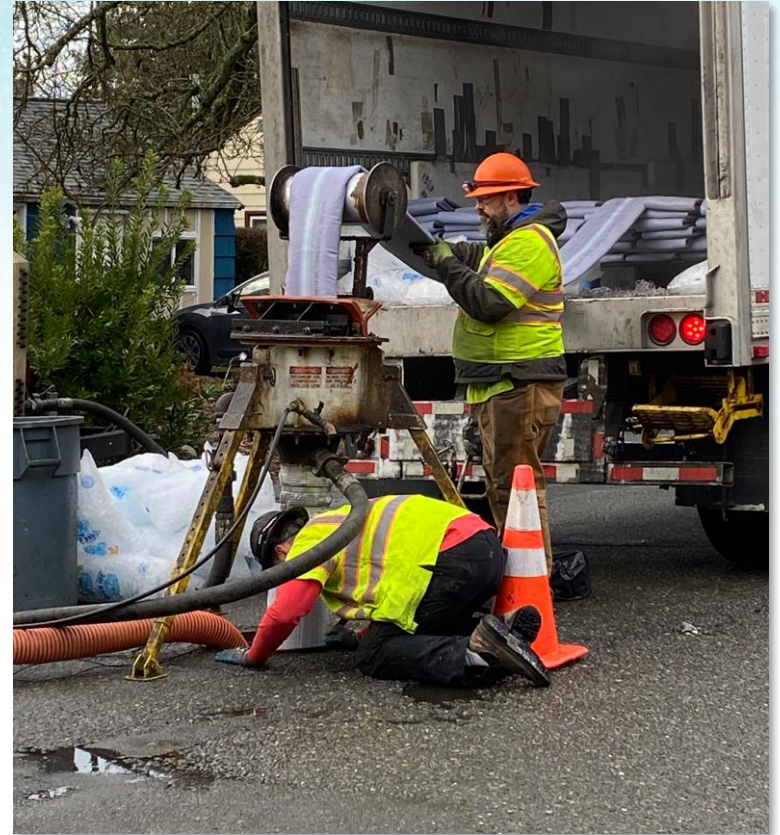
The photo is from SPU's recent Sewer Lining Contract, where Cured-in-Place Pipe (CIPP) lining is being installed.
