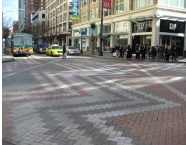
Pine Street Paving at Westlake Park
