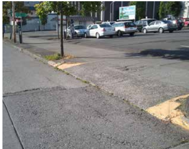
Existing Curb Ramp Conditions
