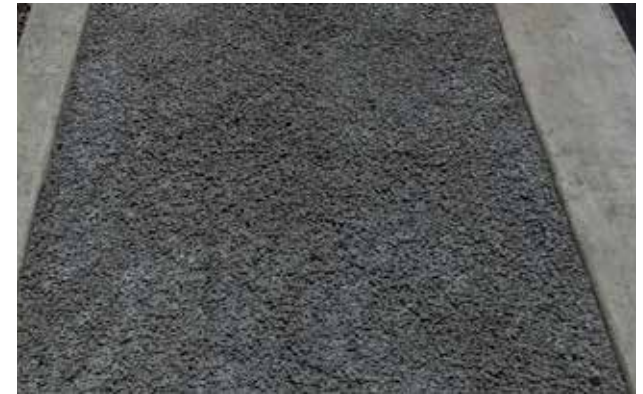
Permeable Concrete Sidewalks
