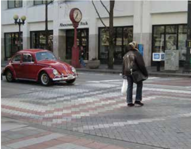
Pine Street Paving at Westlake Park
