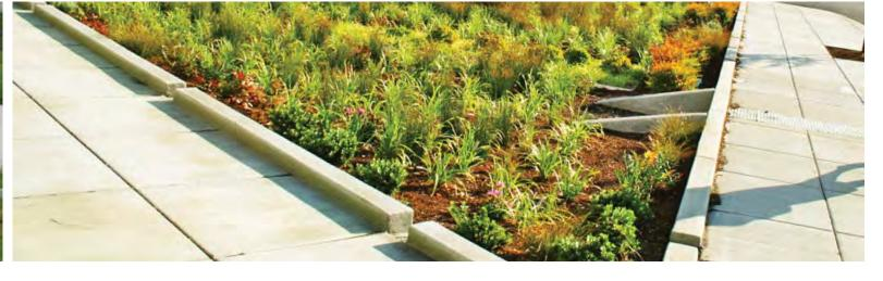
Through the process of bioretention, sediments and contaminants are removed from stormwater using Green Stormwater Infrastructure (GSI) practices such as bioretention ponds, rain gardens and bioswales.
