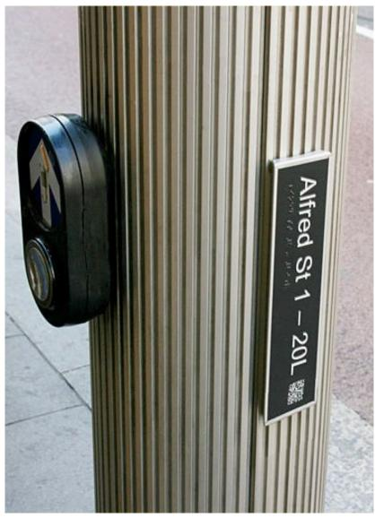
Modern 'street name plate' - Visible, legible, tactile and braille signs at signalized crossings and bus stops?
