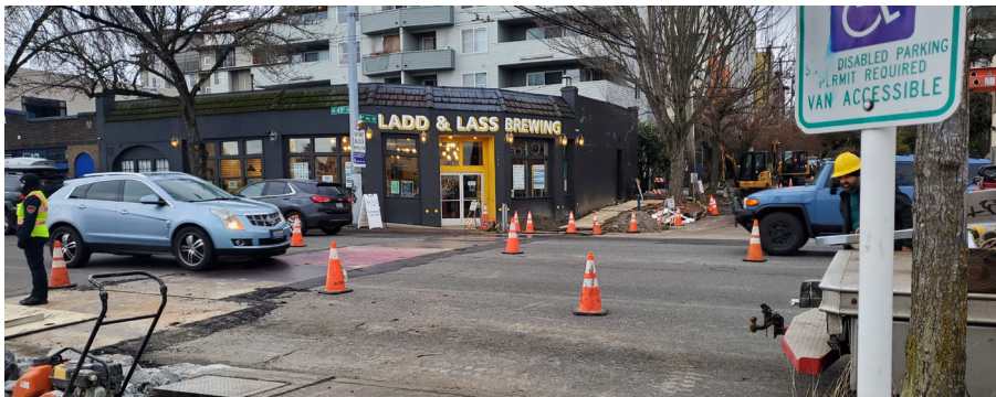
Crews performing work on NE 45th St and 8th Ave NE
