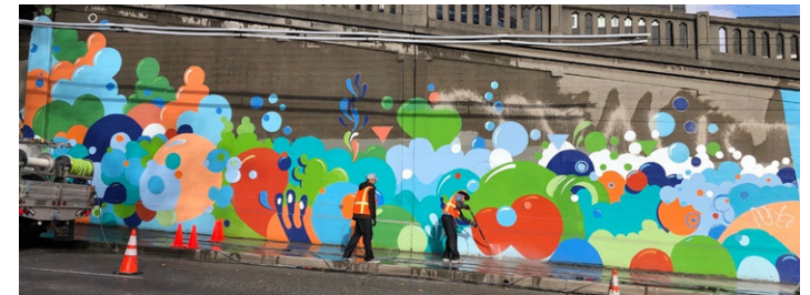
Crews cleaning the mural on N 46th St
