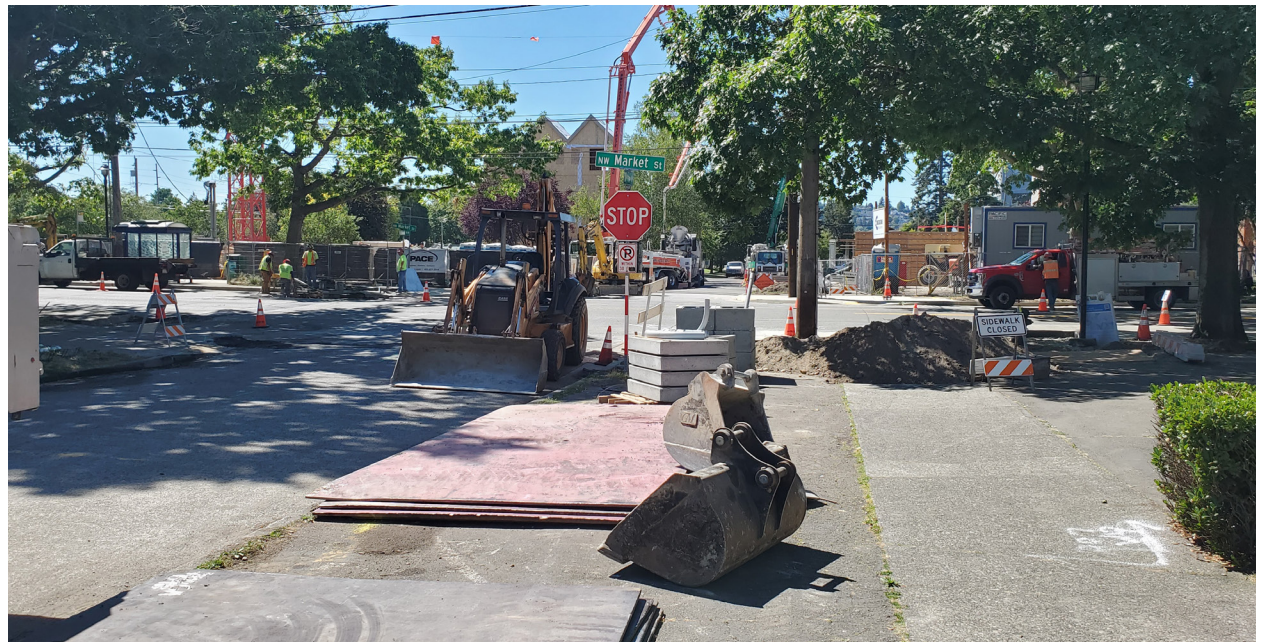
Crews performing work on NW Market St and 11th Ave NW
