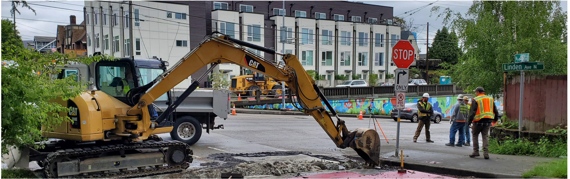
Crews performing work on N 46th St and Linden Ave N
