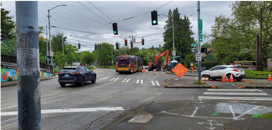
Work underway at N 46th St and Green Lake Way N
