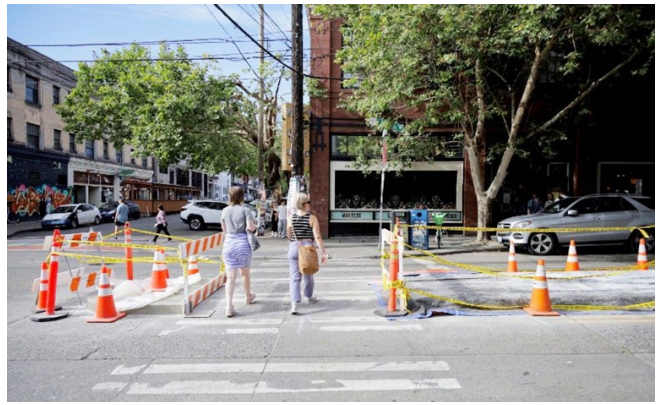
Construction of new island at 10th Ave and E Pike St
