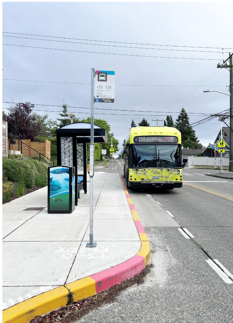
New STM-funded bus stop on 16th Ave SW and SW Thistle.
