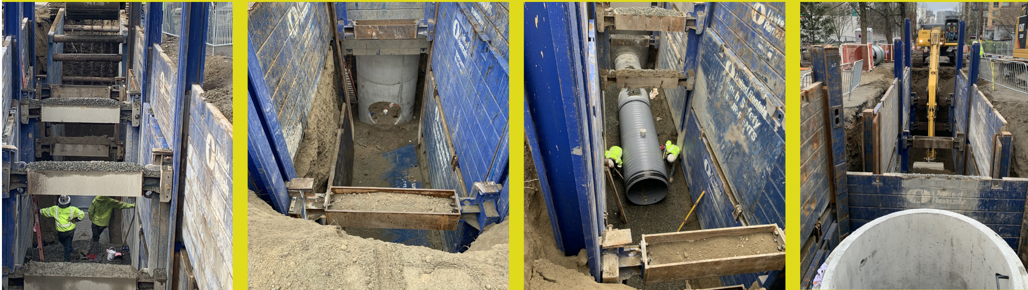
Building the new stormwater tank under E Pine St.
