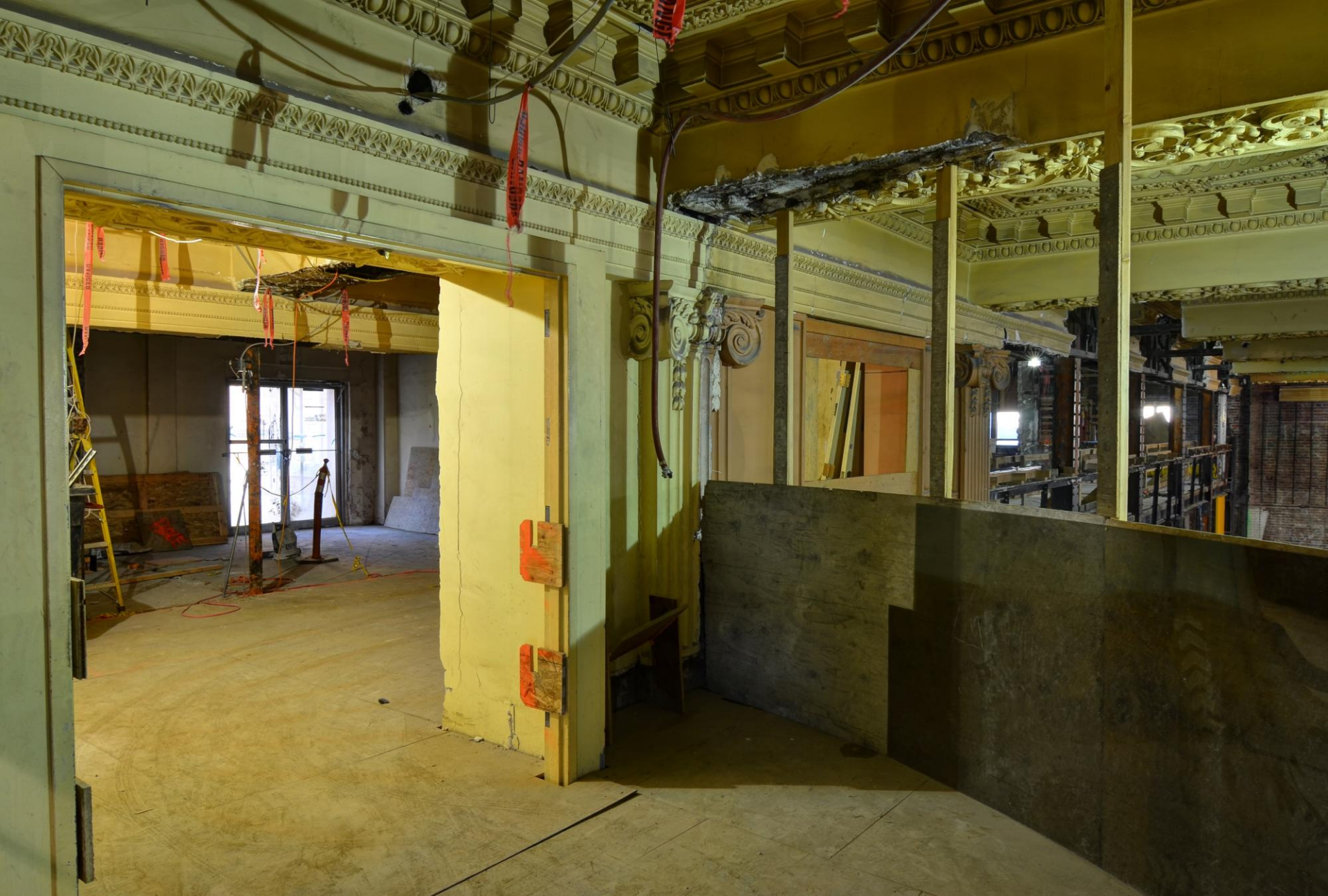
Quarter round balcony as seen from the 2 nd level. All damaged ornamental plaster will be repaired or replaced.
