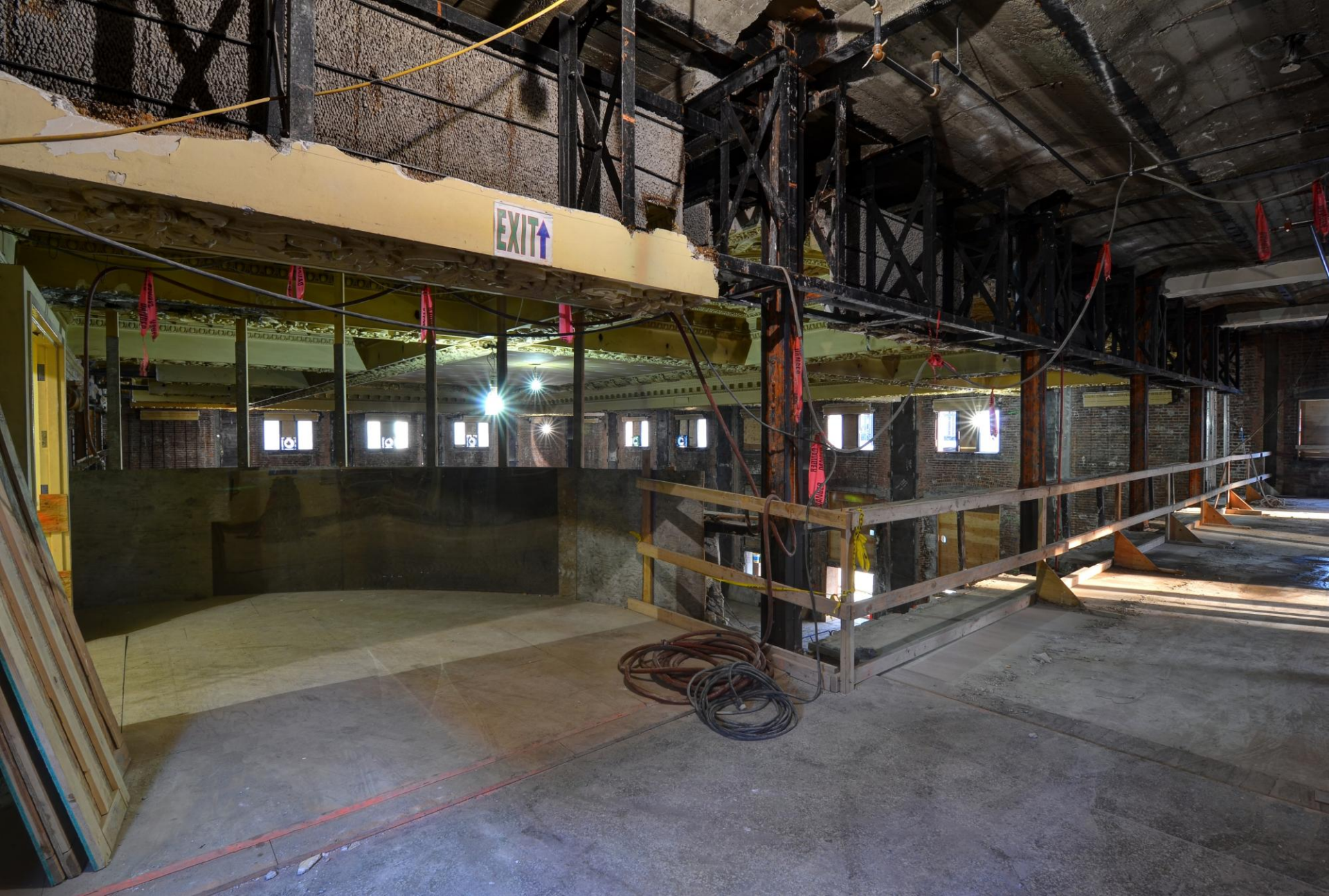
Part of the 2nd level corridor will be opened to the public to view of the waiting room below. Original steel trusses have been exposed for inspection prior to construction.
