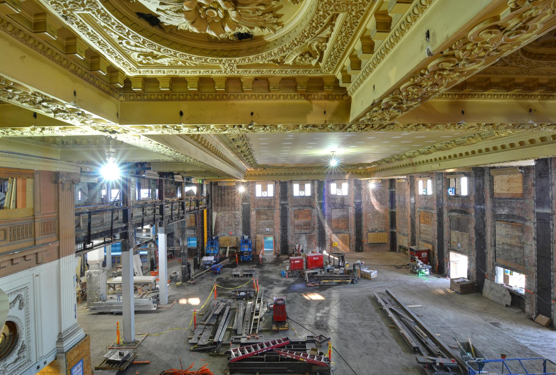
Holes and cracks in the ornamental plaster ceiling are currently being patched and repaired. Plaster molds are made and casted right on site.
