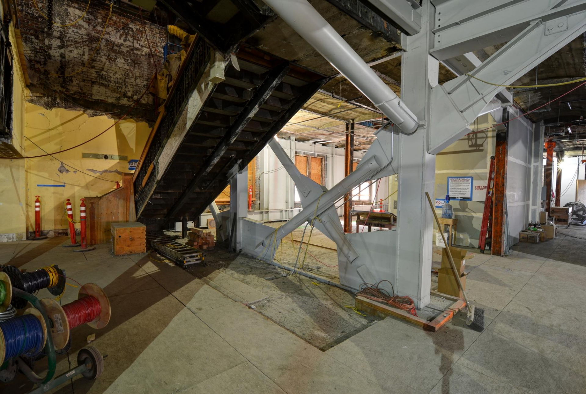
Massive new steel trusses have been installed as part of the seismic upgrade system to counter the weight of the tower.
