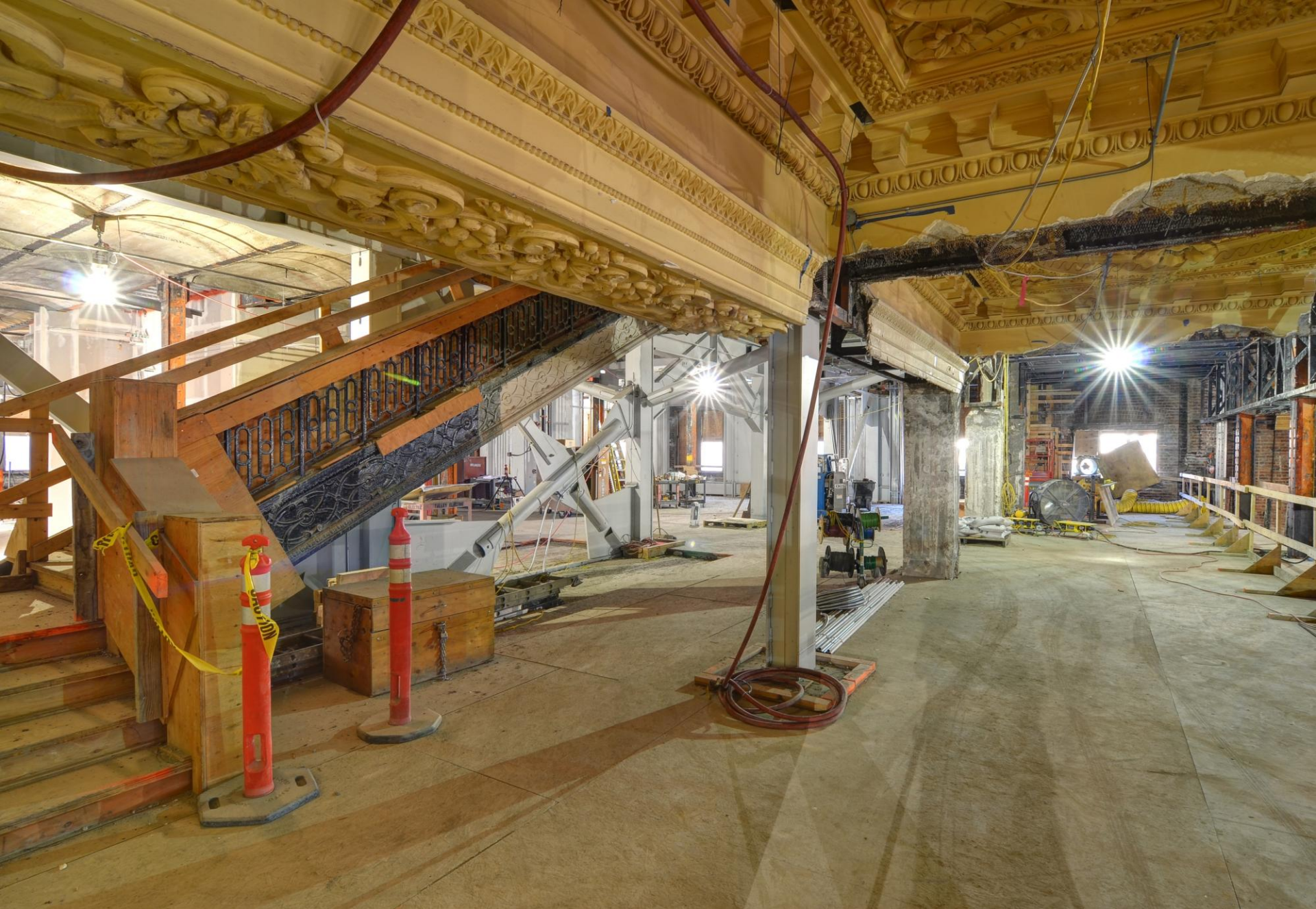
The terrazzo floor is protected by plywood sheathing. All interior partition have been removed.
