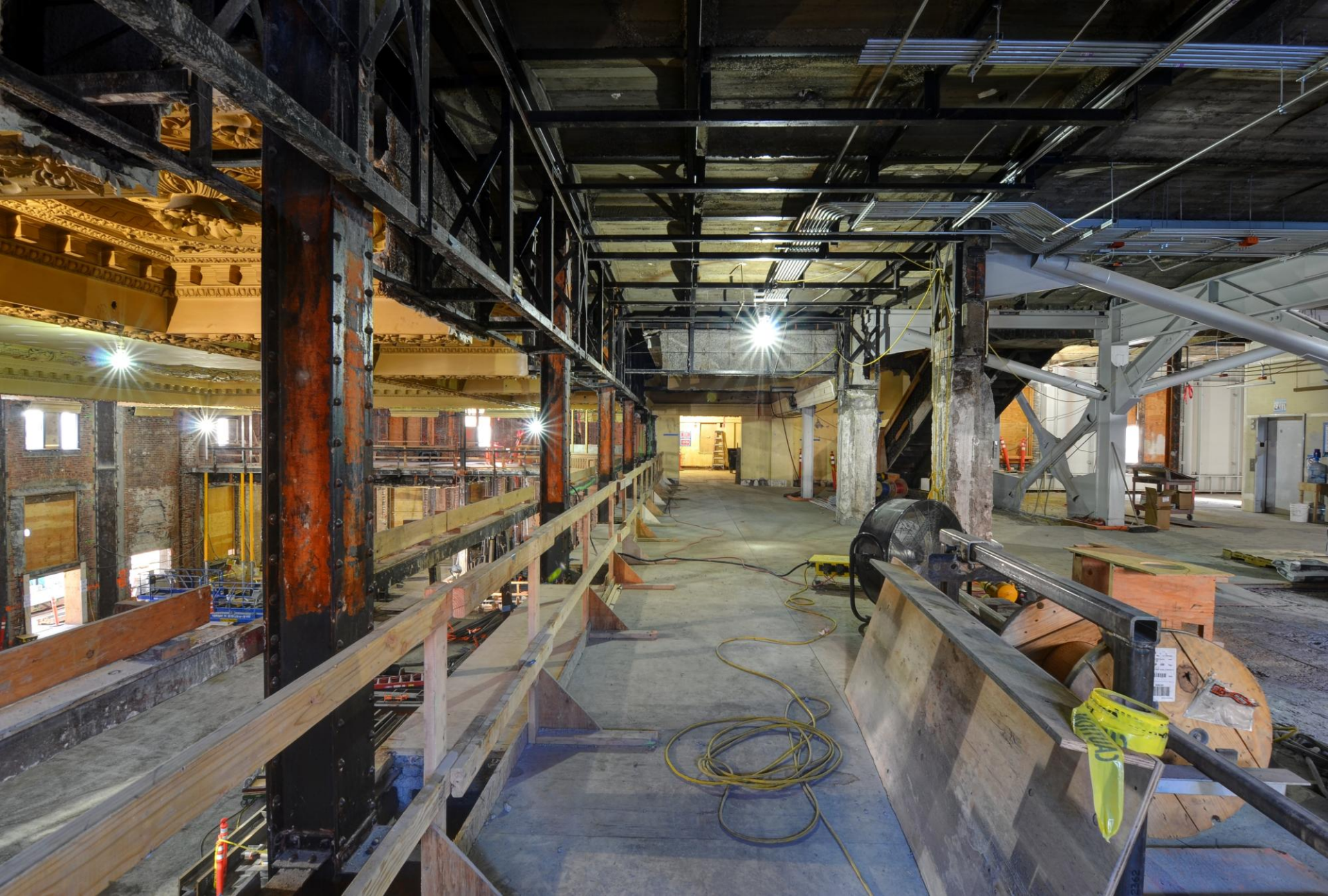
From the east wall looking west along the 2 nd level balcony. Some plaster on this level has been removed for seismic upgrade.
