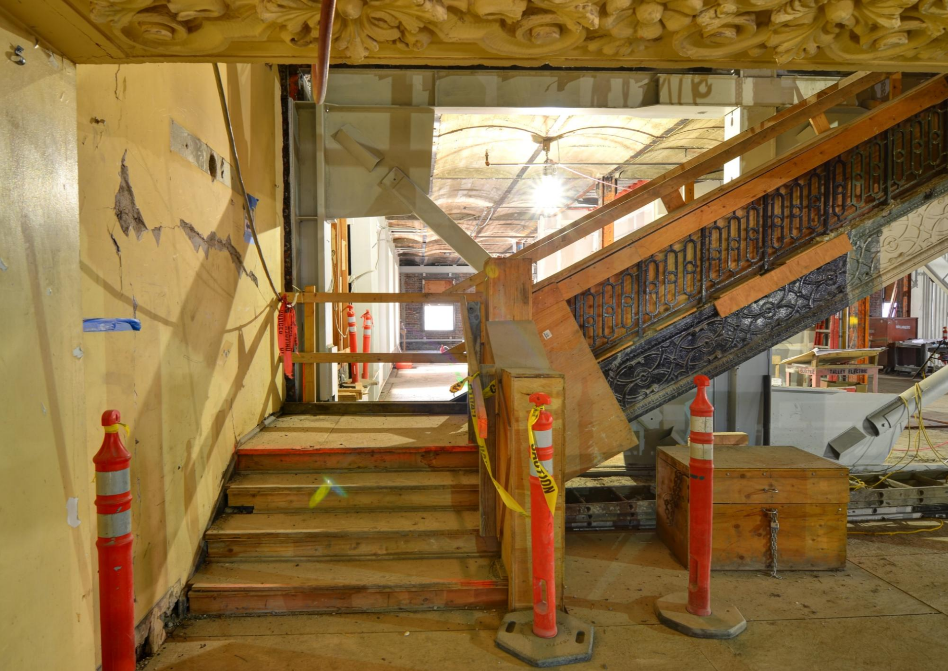
The original historic stairs are also protected by plywood from accidental construction damage.
