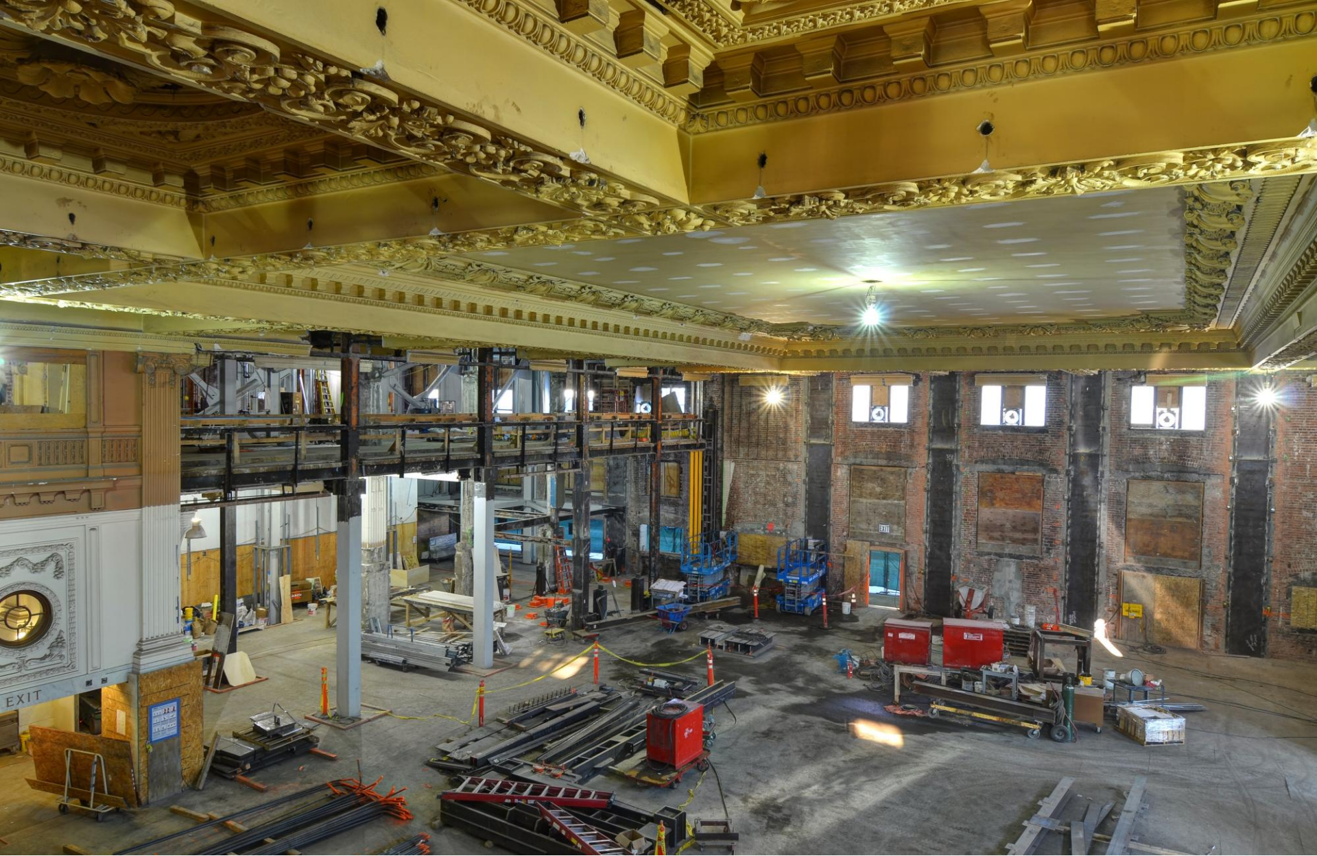
An acoustical ceiling that covered the 2 nd floor windows as well as the balcony was installed at the station in the 1960s as part of a “modernization” effort. Holes in the ornamental plaster ceiling are results of this decision.
