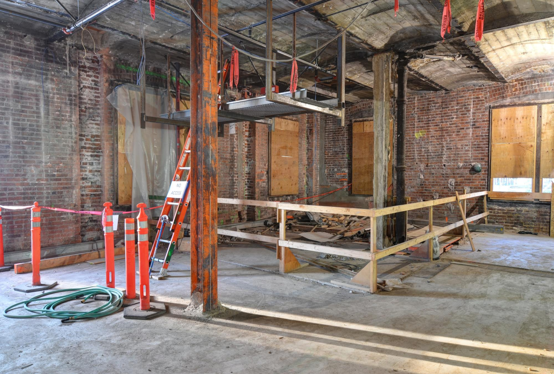
A view of the exposed brick walls of an upper floor. All windows have been removed for off site restoration.
