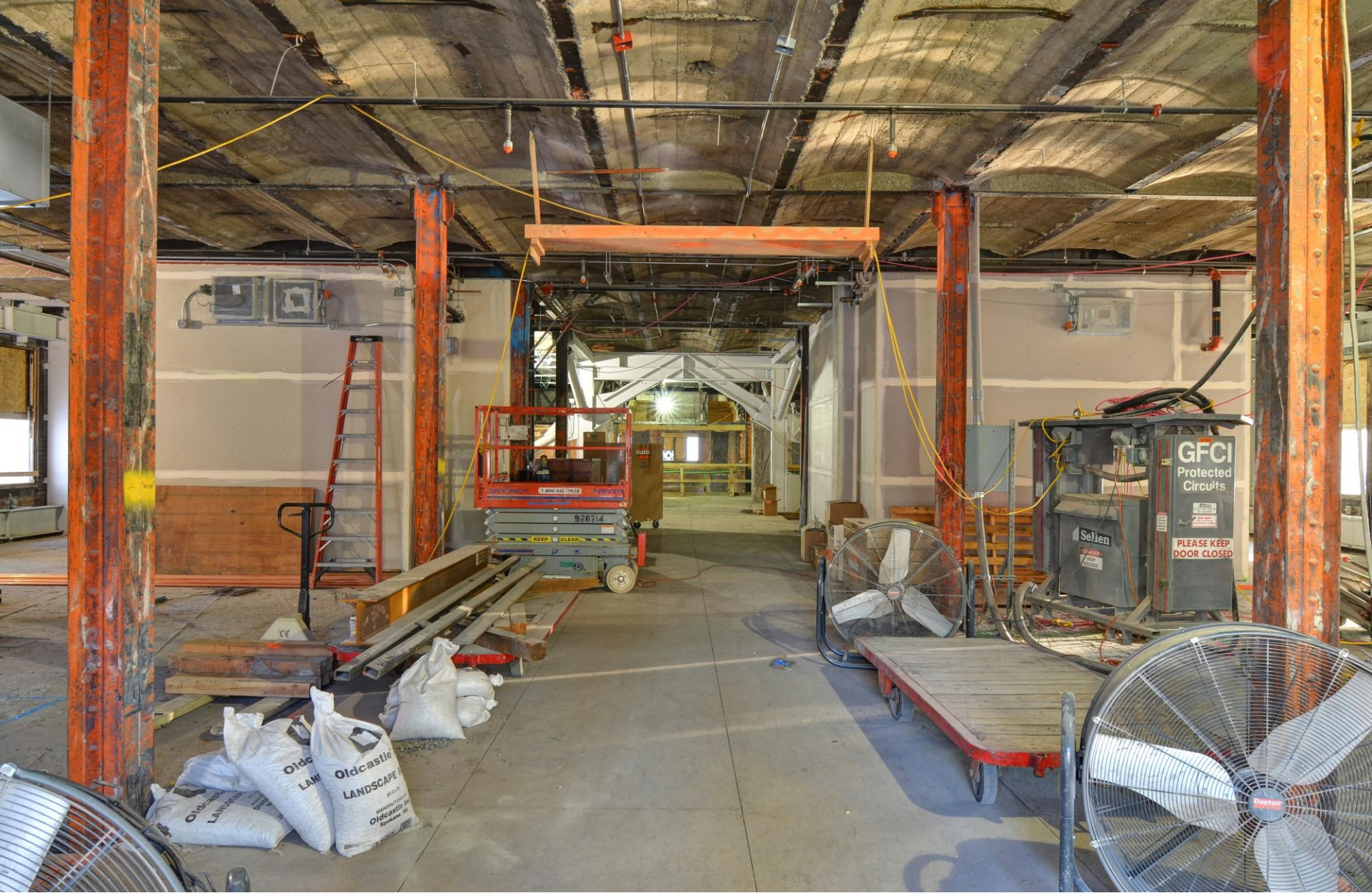
2 nd level looking south at the new stair well(left) and elevator(right). The stair well will connect the 3 rd floor to the 2 nd floor, and the elevator connects the terminal level to both 2 nd and 3 rd floors. Elevator installation has been completed but the stair well is still under construction.
