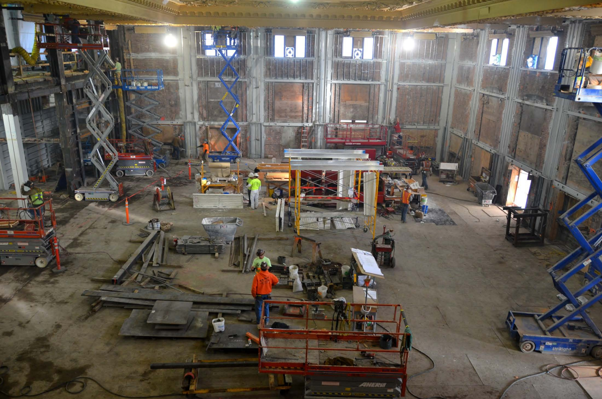
Seismic steel trusses were installed over new white columns for additional load bearings. New ornamental plaster walls will hide these new structural steel reinforcement.
