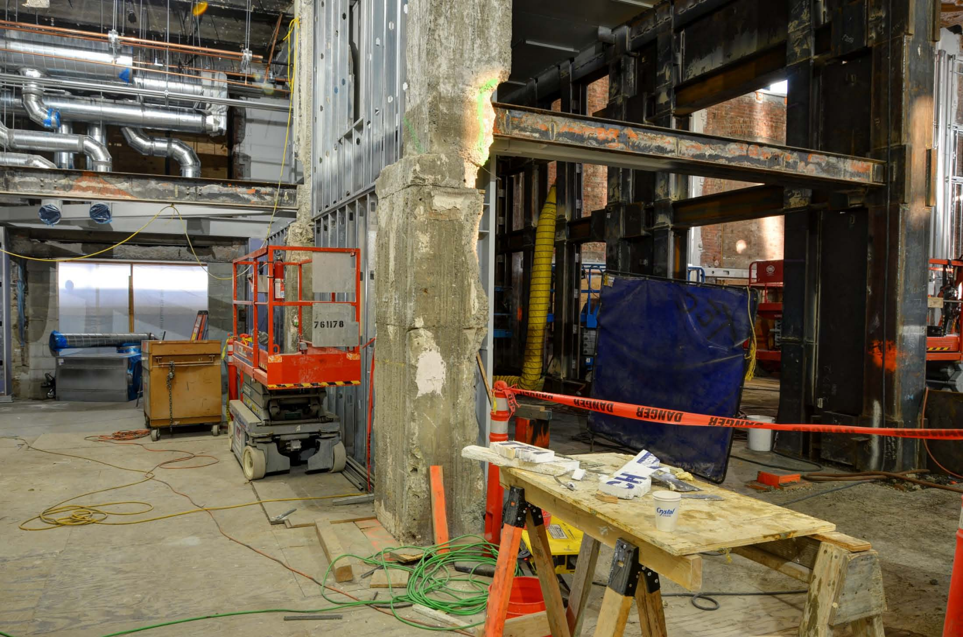
HVAC was installed at the previous electrical room and Amtrak cafeteria located along the east trackside perimeter. This area will be the future Men's restroom. Two new double doors will be installed for access and egress. One of the new double door location is shown in the photo.
