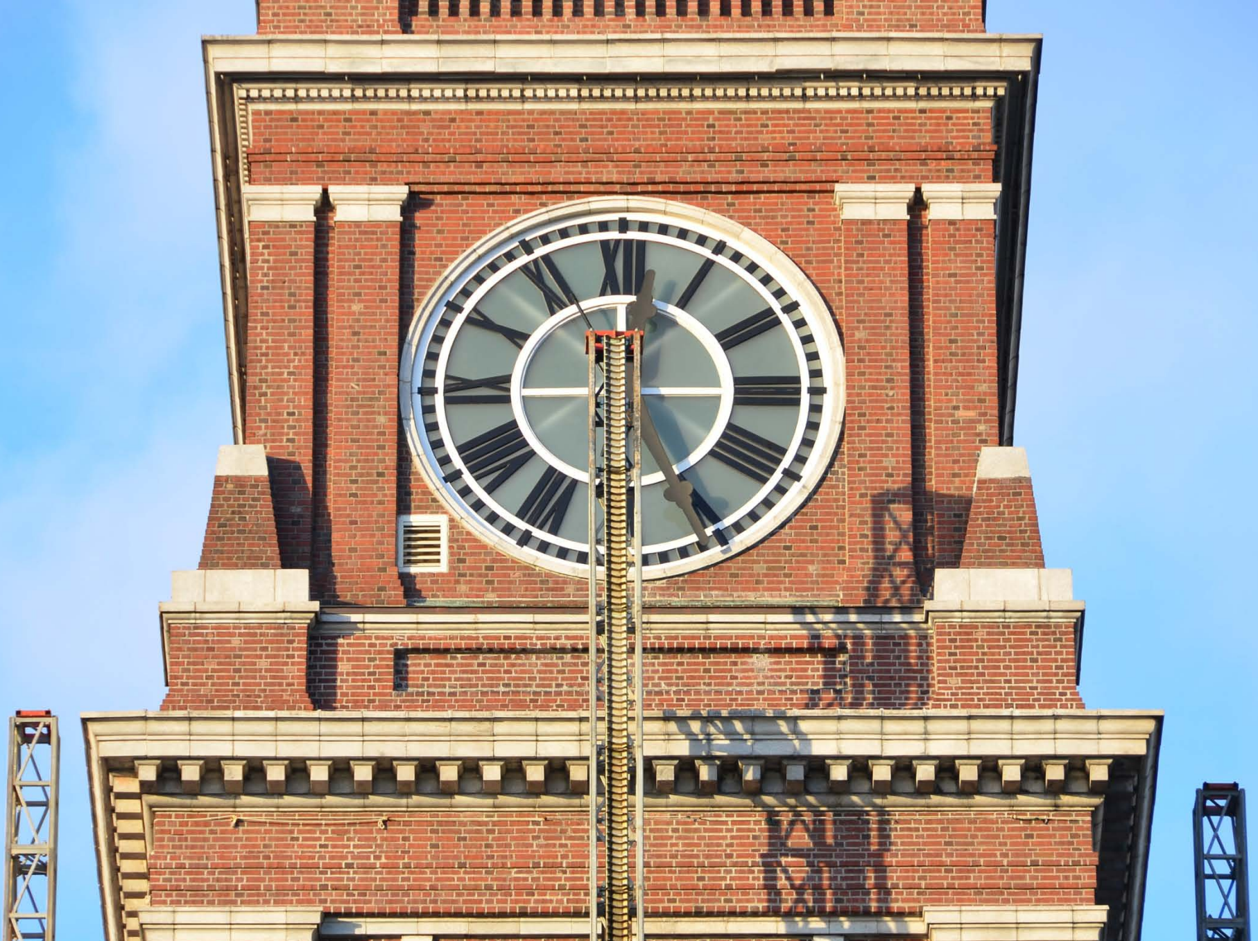
Terracotta dental trim repaired. All new anchorage attachments are stainless steel for longevity.
