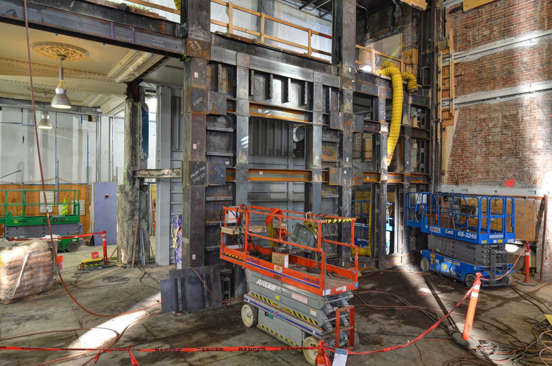
Steel shear wall shown is installed over a 15'X30' mat foundation, deep driven piles and is also tied to the exterior 4'X4' ring beam.
