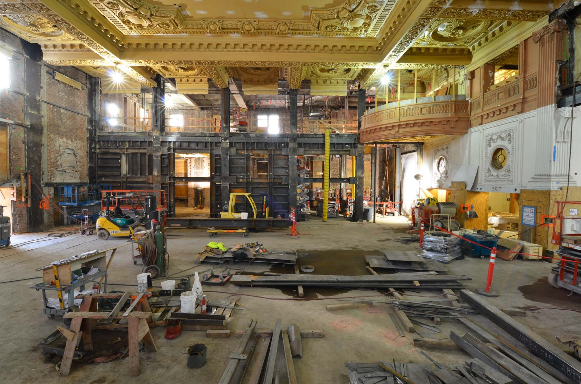
Massive steel shear wall shown is tied to the 30'X30' mat foundation and 46' deep piles below for structural rigidity.
