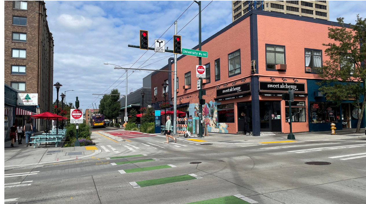
Example of bike and transit treatments at NE 43 rd St and University Way NE
