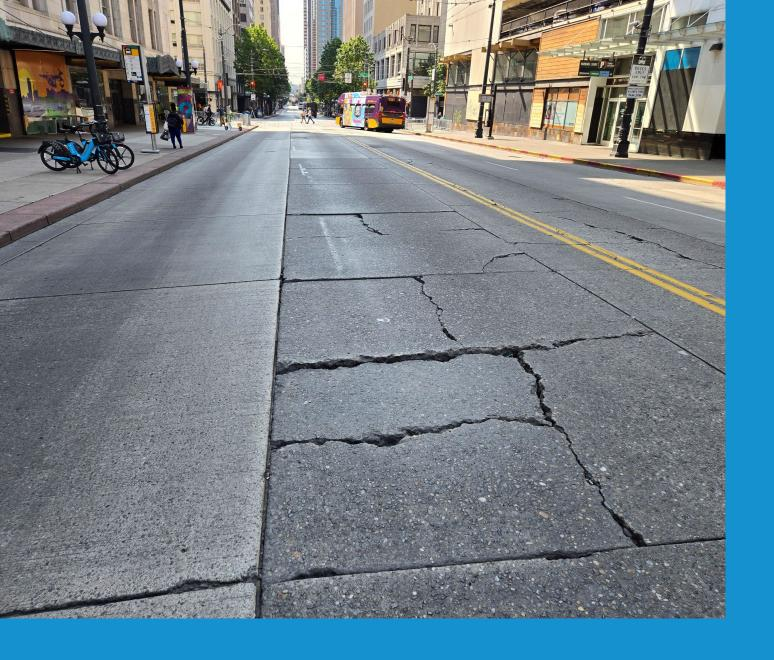
Several concrete panels are cracked into multiple pieces
