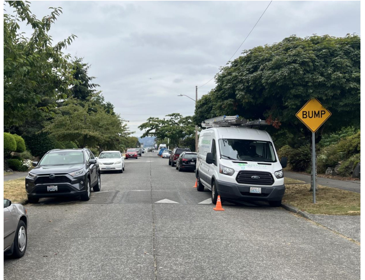
Speed cushion on 13th Ave S
