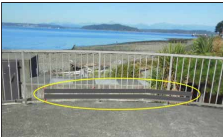
Conceptual view showing the approximate location of the conduits. Conduits will be on the water side of the railing.
