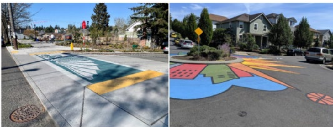
Traffic calming elements on Neighborhood Greenways could include raised crosswalks (left) and traffic circles (right).
