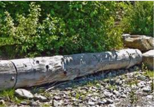
Large Salvaged Logs Seating and Stabilization
