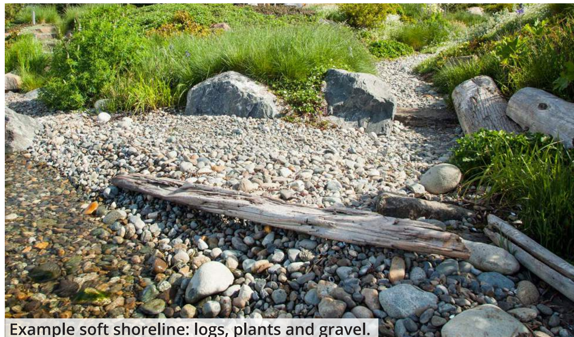
Log reinforcement and gravel on Seattle shoreline.
