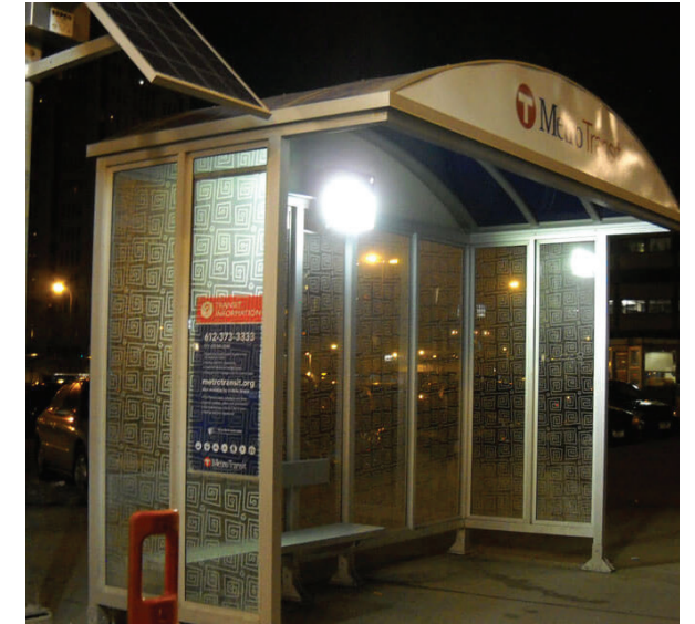
C Transit stop lighting
