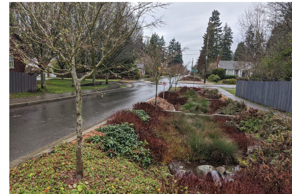
B Green stormwater infrastructure
