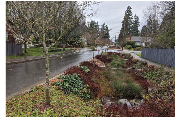
B Green stormwater infrastructure
