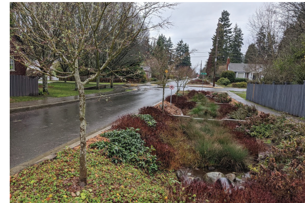
B Green stormwater infrastructure
