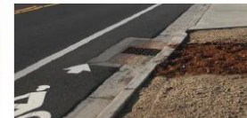
Upgrade drainage in spot locations.
