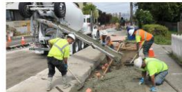
Pave with new concrete.
