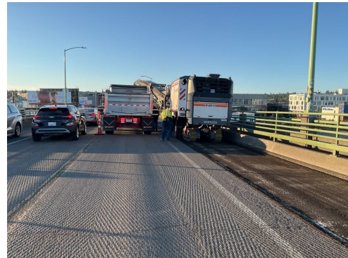
Example of road surface that has been ground down.
