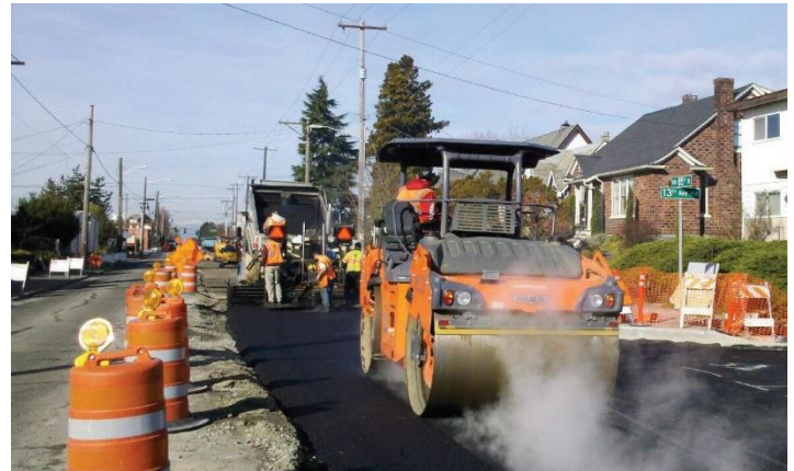
Example of crews paving a street
