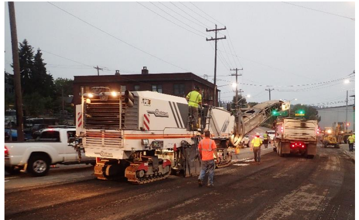
Example of crews grinding the street
