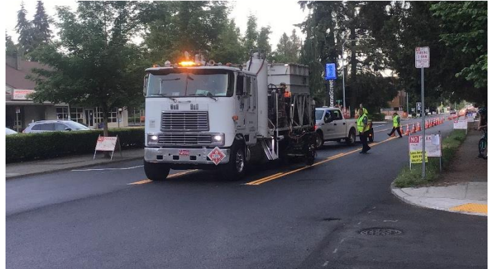
Example of crews striping the street
