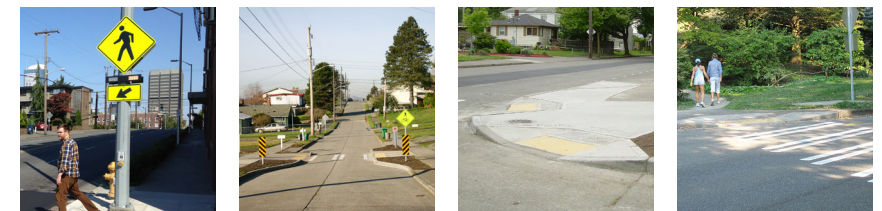
1 Crossing beacon 2 Curb bulb 3 Curb ramp 4 Crosswalk
