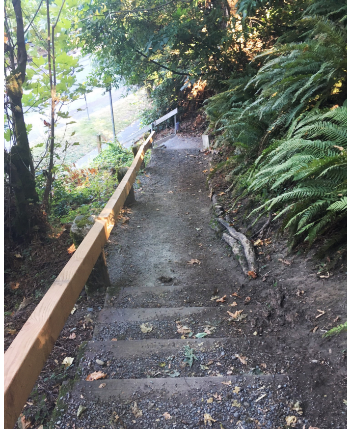
Existing stairway. Improvements are planned for the stairway at Interlaken Park near Boyer Ave E and E Howe St in summer 2018.
