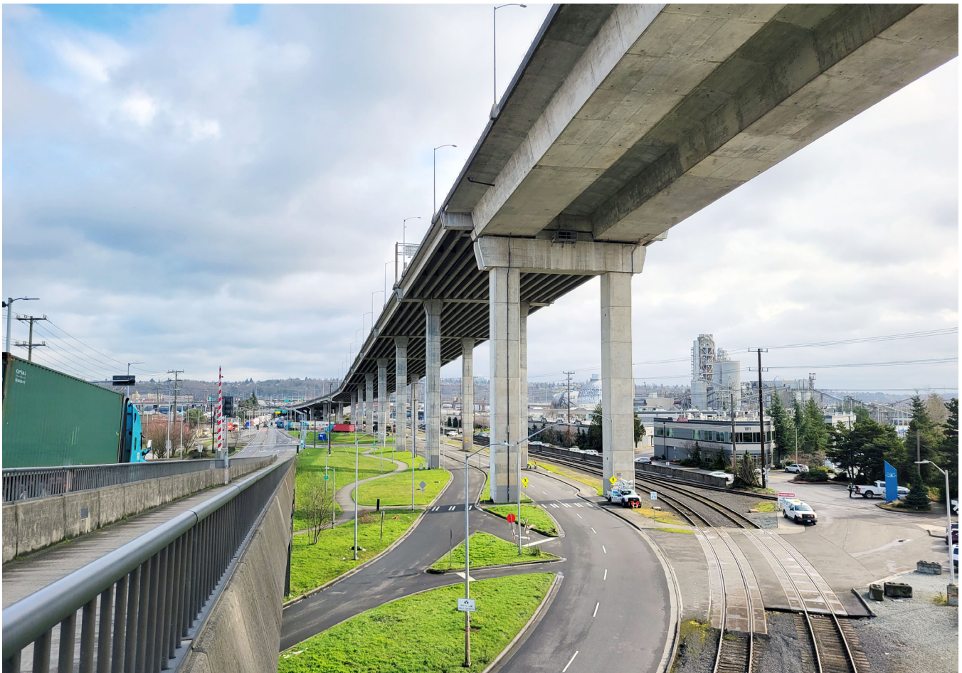
West Seattle High-Rise Bridge and Spokane St Swing Bridge
