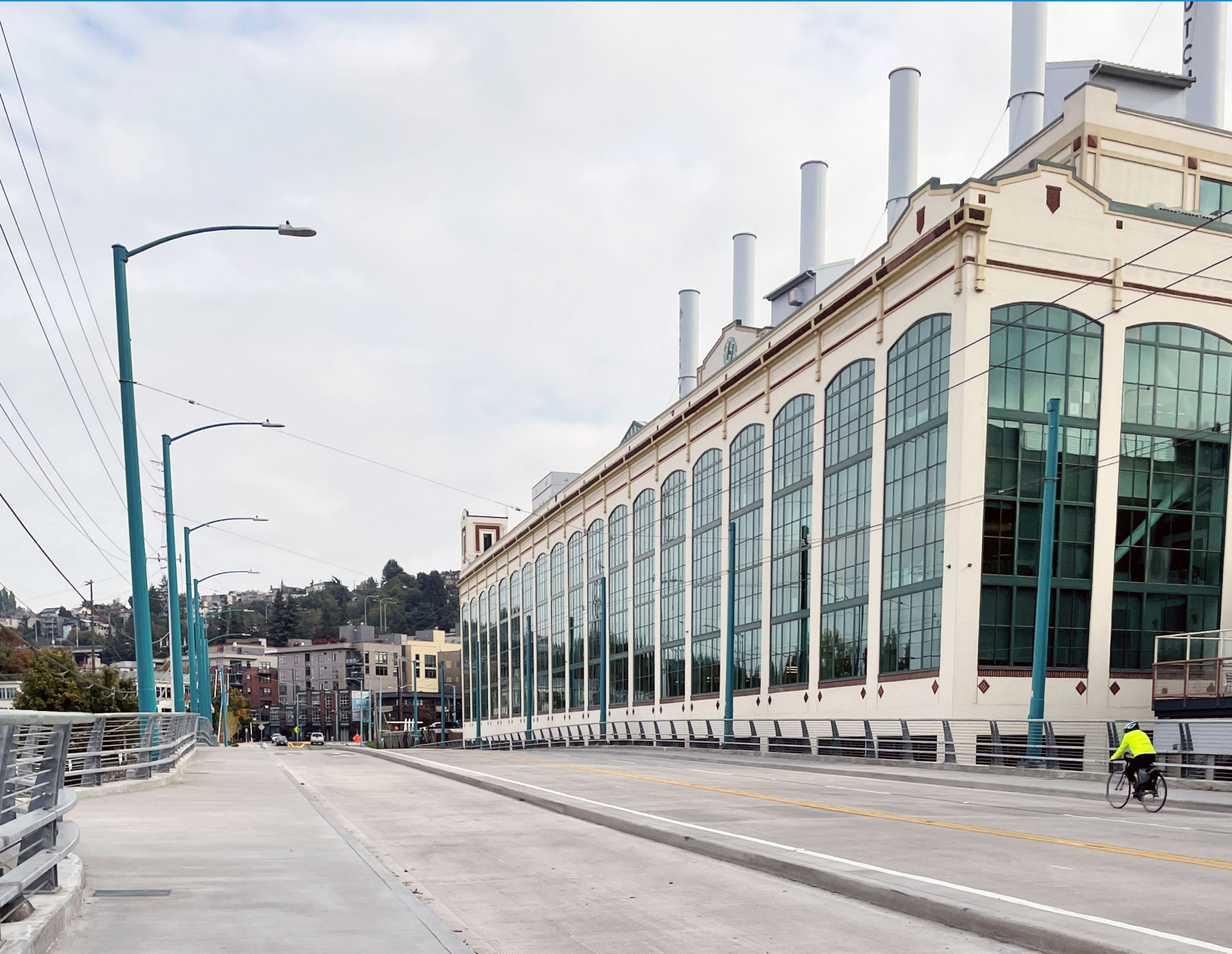
Fairview Ave N Bridge
