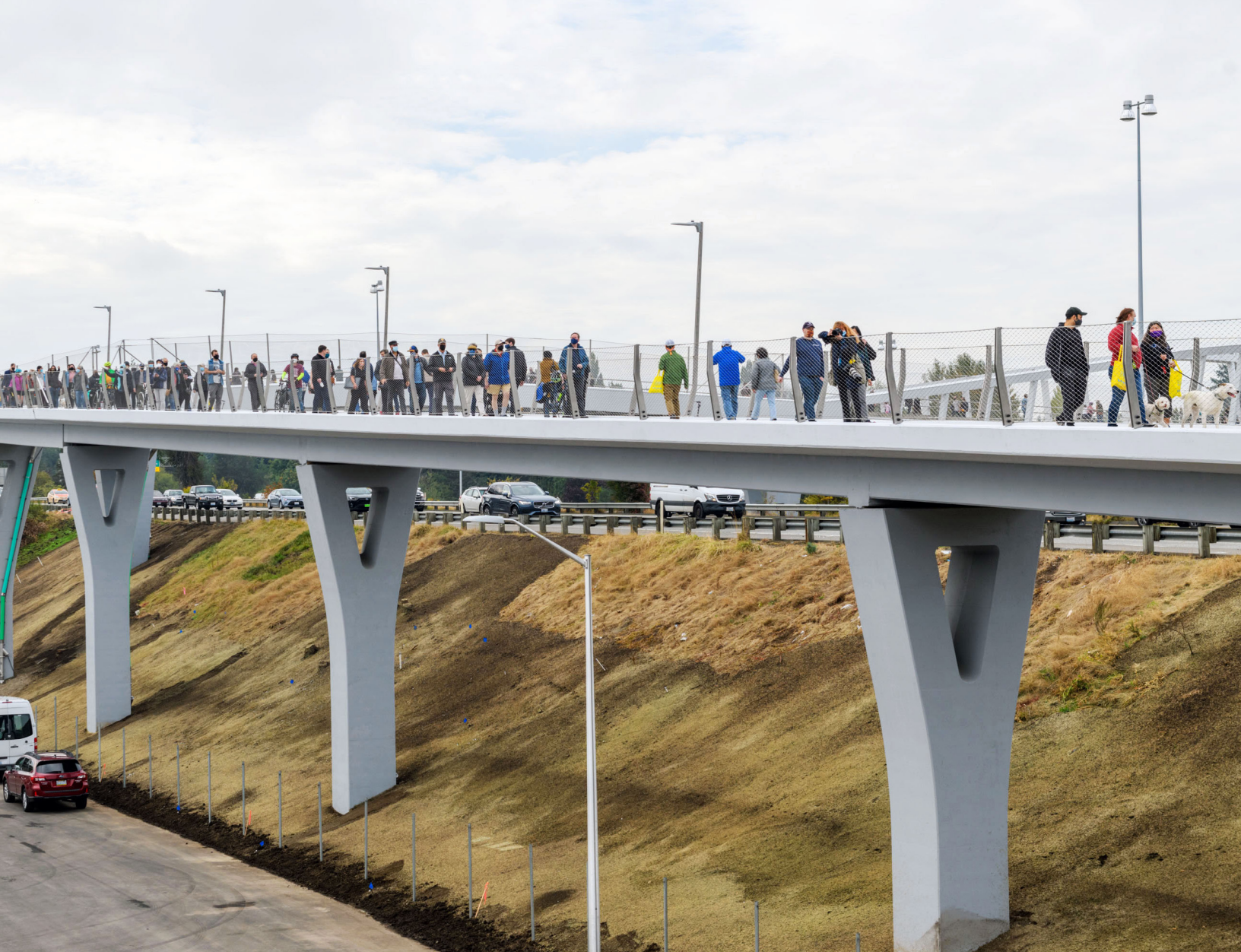
John Lewis Memorial Bridge
