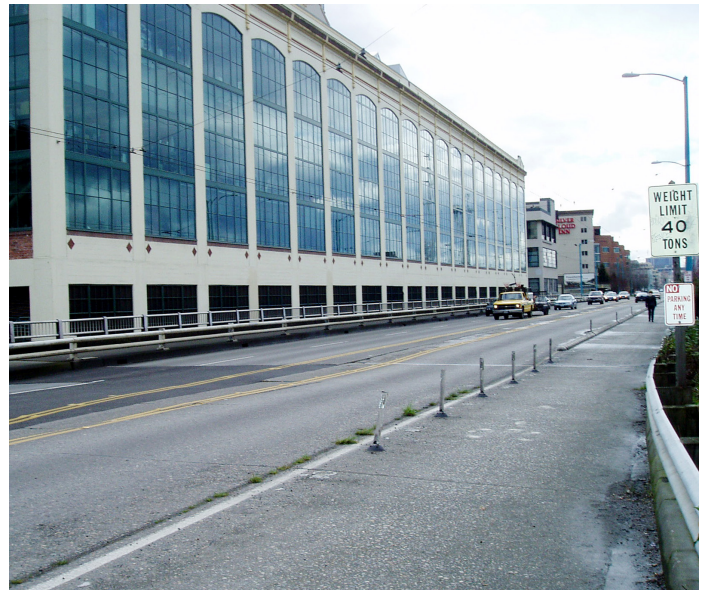
Fairview Ave N bridge directly next to the historic Lake Union Steam Plant Building (currently Zymogenetics).
