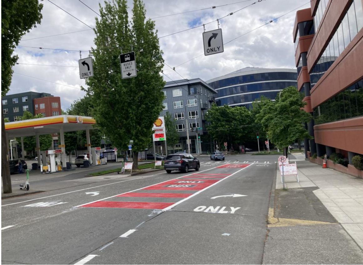
Looking South: New Bus-only Turn Lane on Queen Anne Ave N
