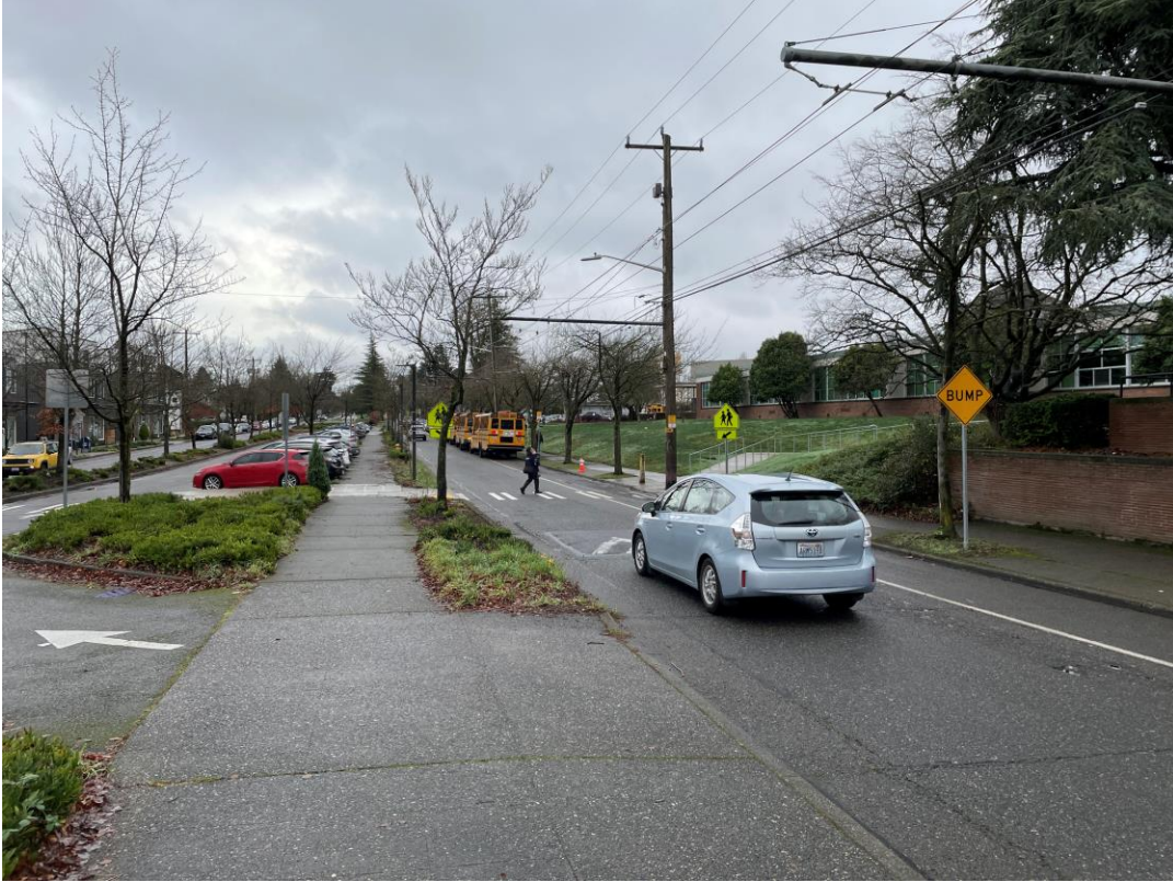
Beacon Ave S at the Van Asselt School Interim Site, facing south.
