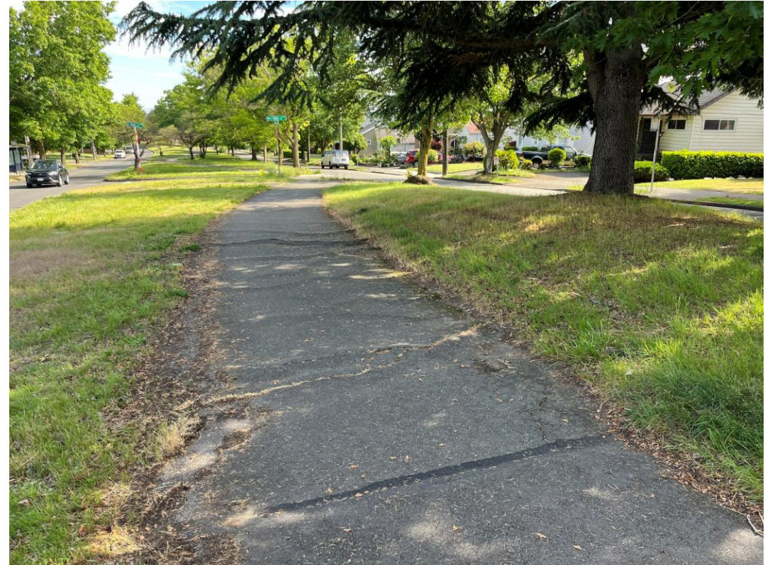
Beacon Ave multi-use path pavement near S Holly St, facing south.
