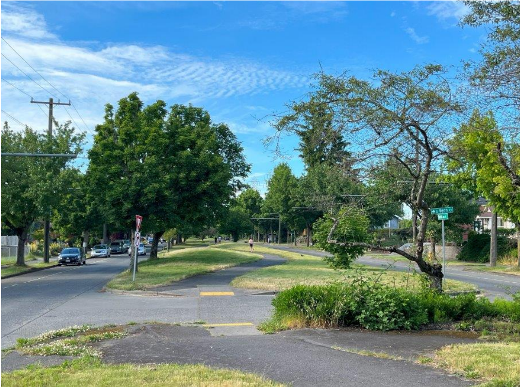
Beacon Ave S multi-use path near S Vern St, facing north.
