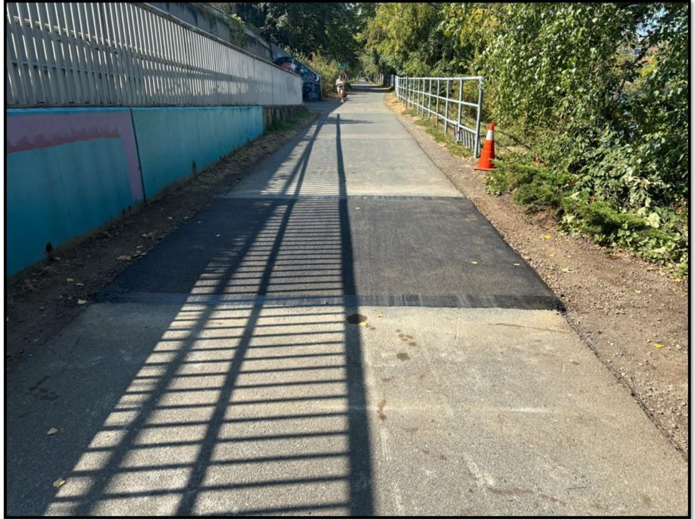
Recent repair along Ship Canal Trail
