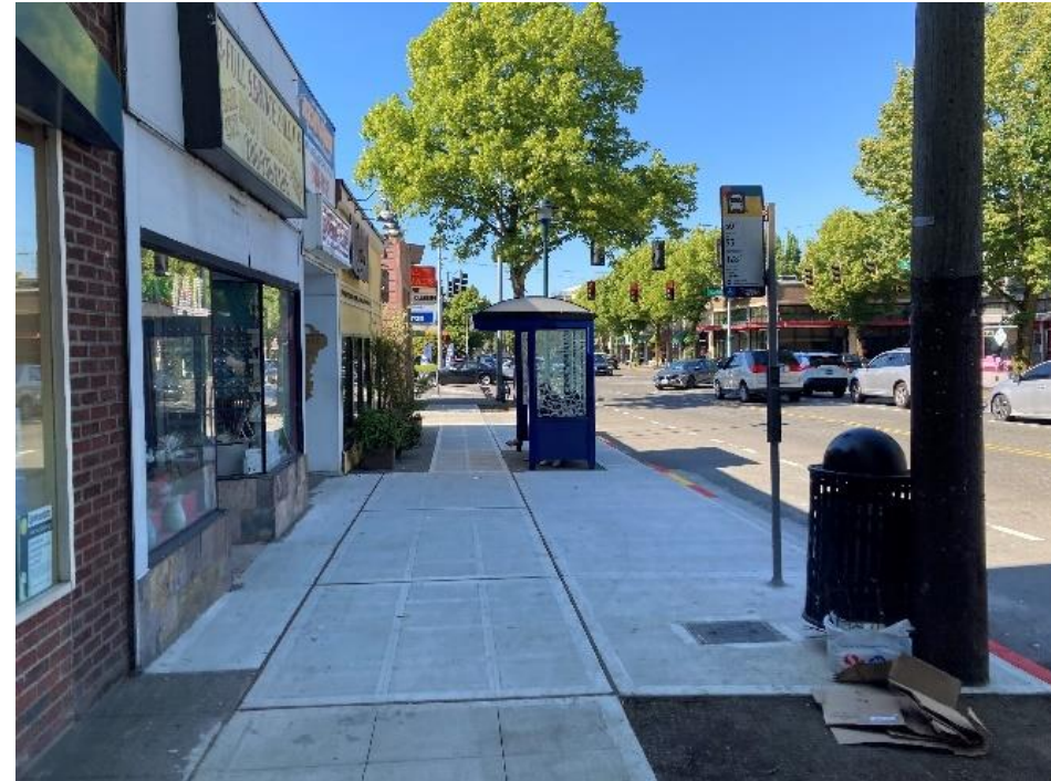
Repaired and improved bus zone on California Ave SW and Admiral Way N.
