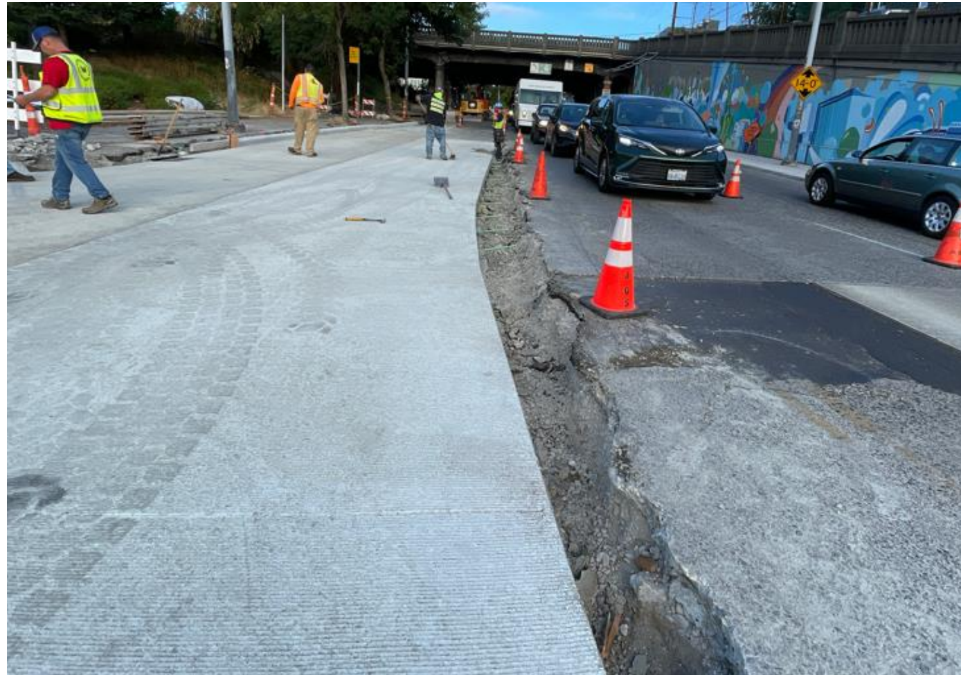
Repaving on N 46th St
