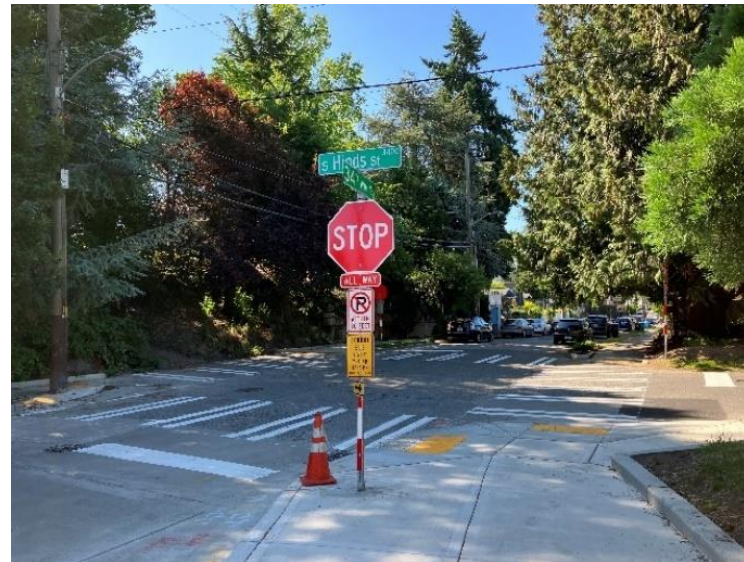
One of three new all-way stops near John Muir Elementary School
