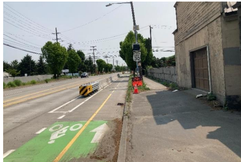
New protected bike lane on West Marginal Way
