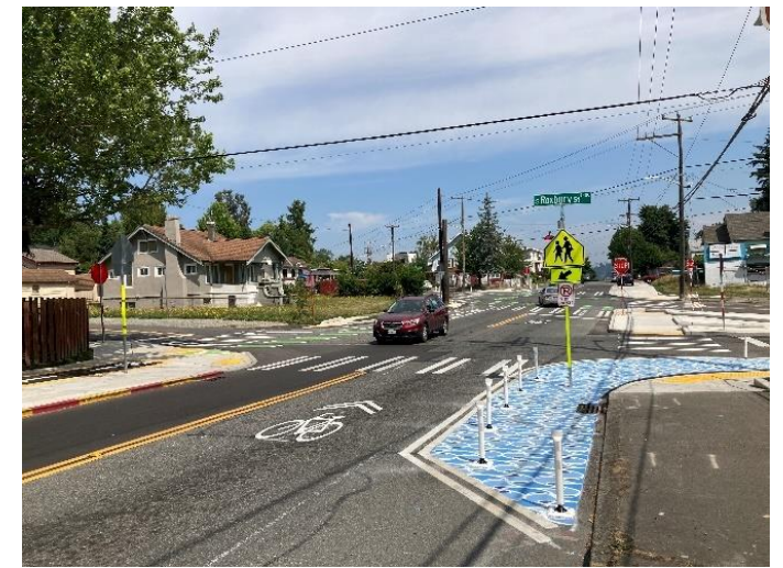
51st Ave S and Renton Ave S Traffic Safety Enhancements project
