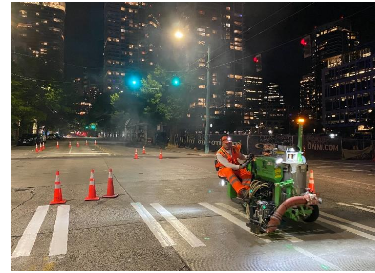
Crosswalk remarking on Fairview Ave E
