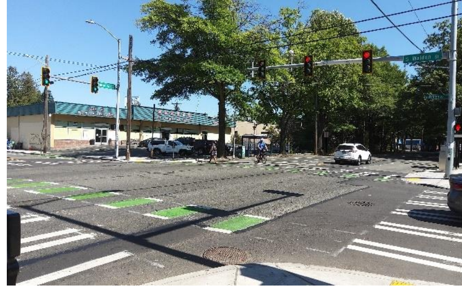
Improved crossings on Rainier Ave S as part of Route 7 work.
