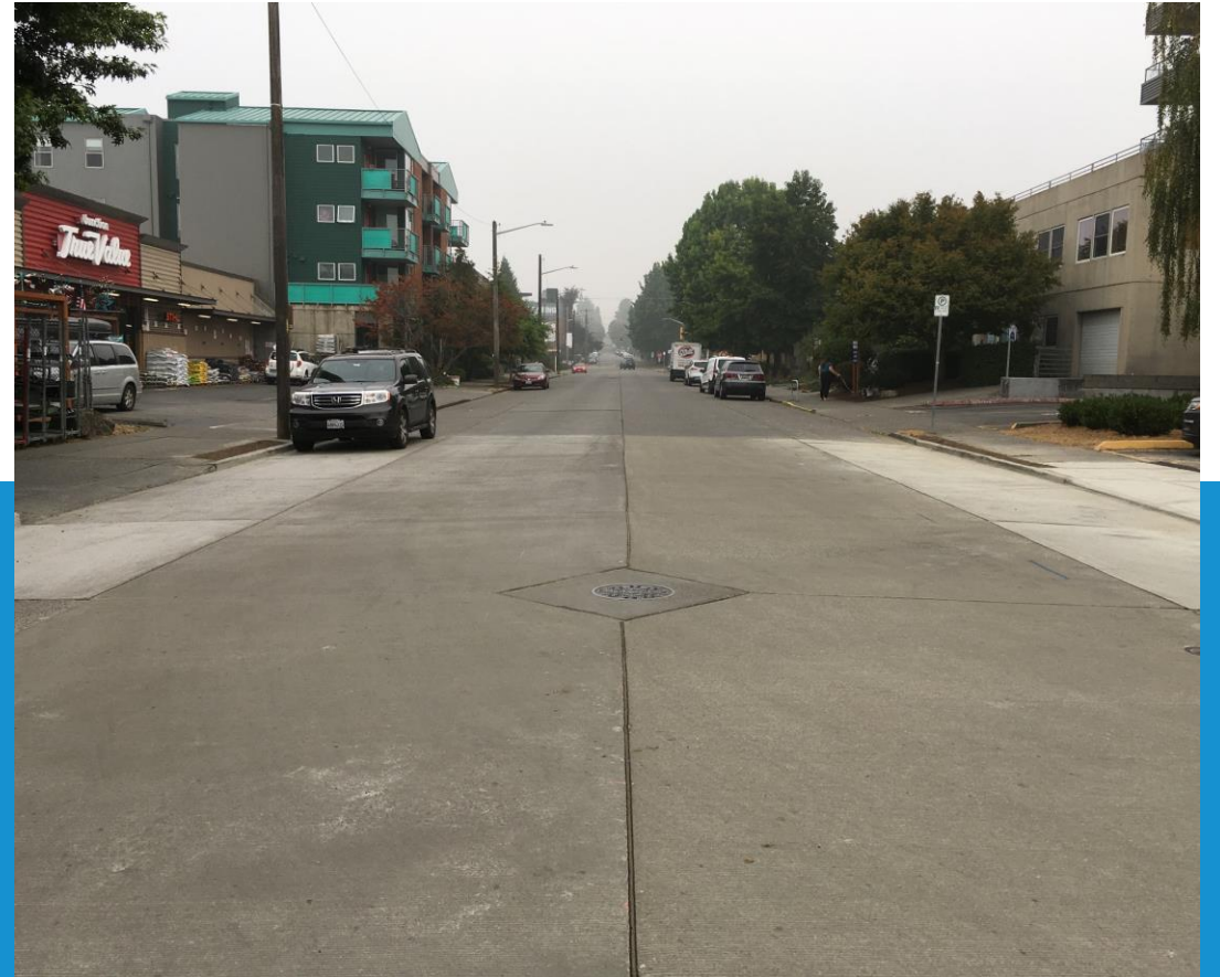
44 th Ave SW - After
