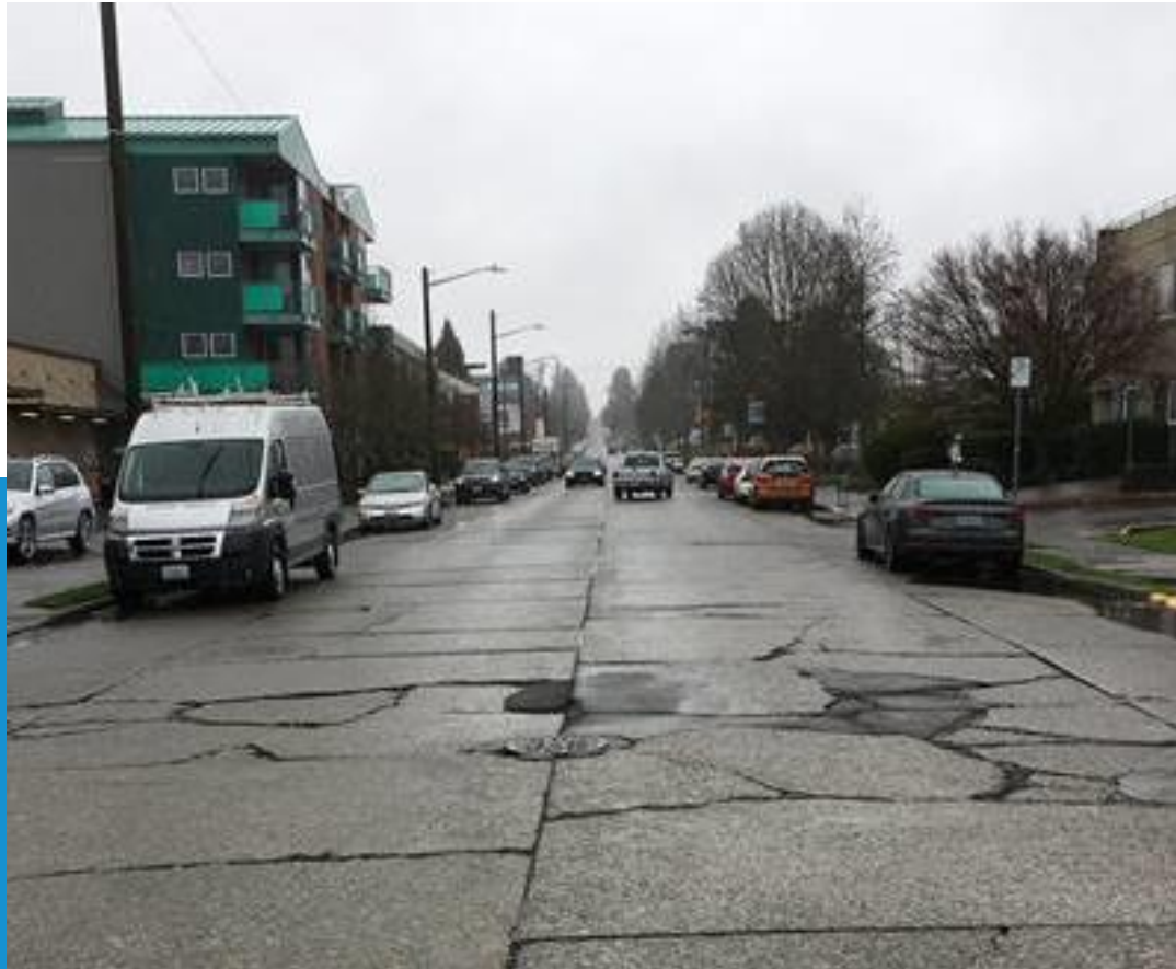
44 th Ave SW - Before
