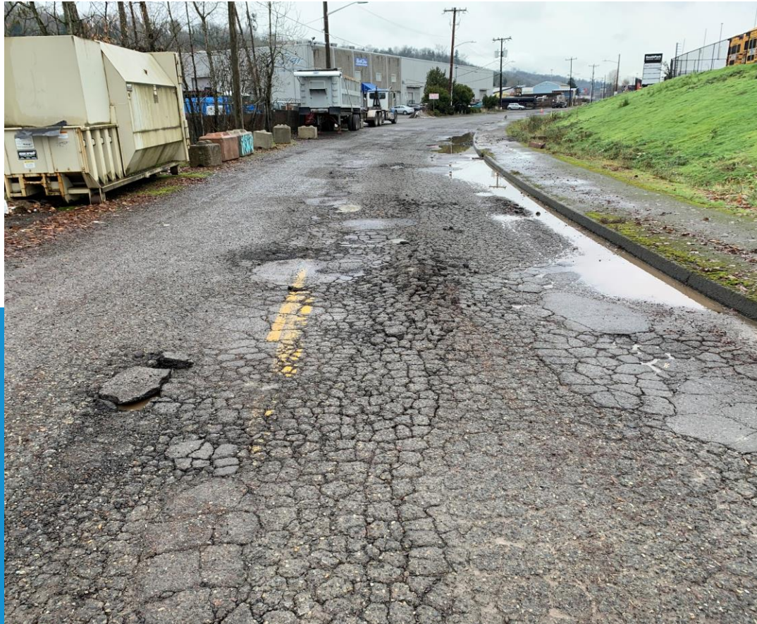
Occidental Ave S - Before
