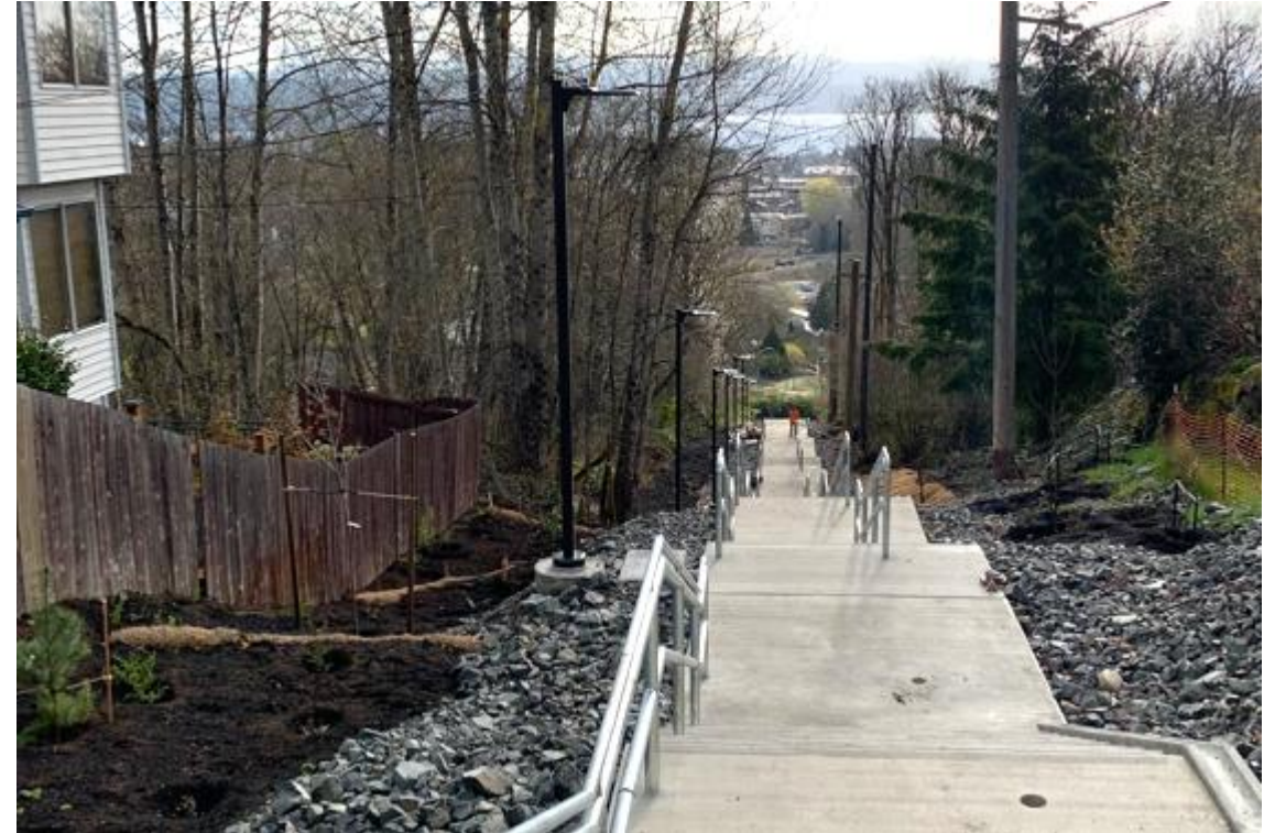
New stairway at S Henderson St.
