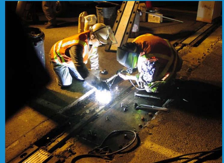
Expansion joint repair on University Bridge
