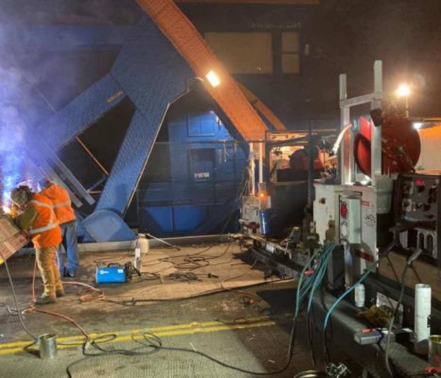
Deck welding repairs on the Fremont Bridge.
