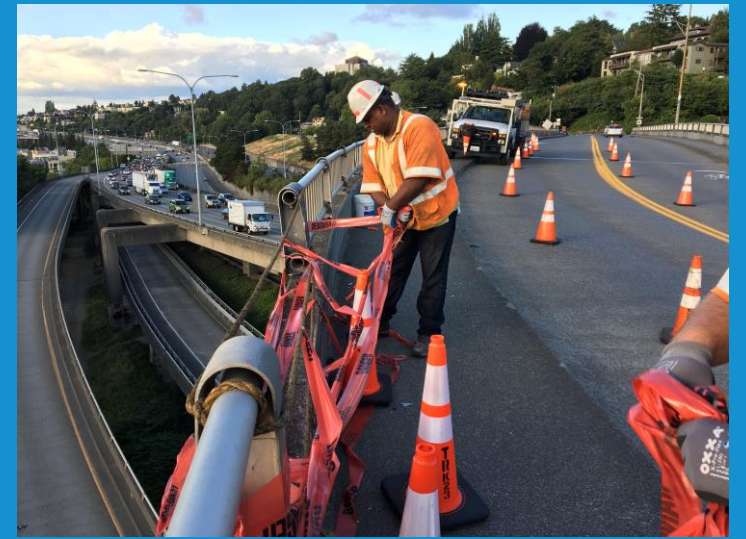
Rail repairs on Lakeview Blvd E Bridge
