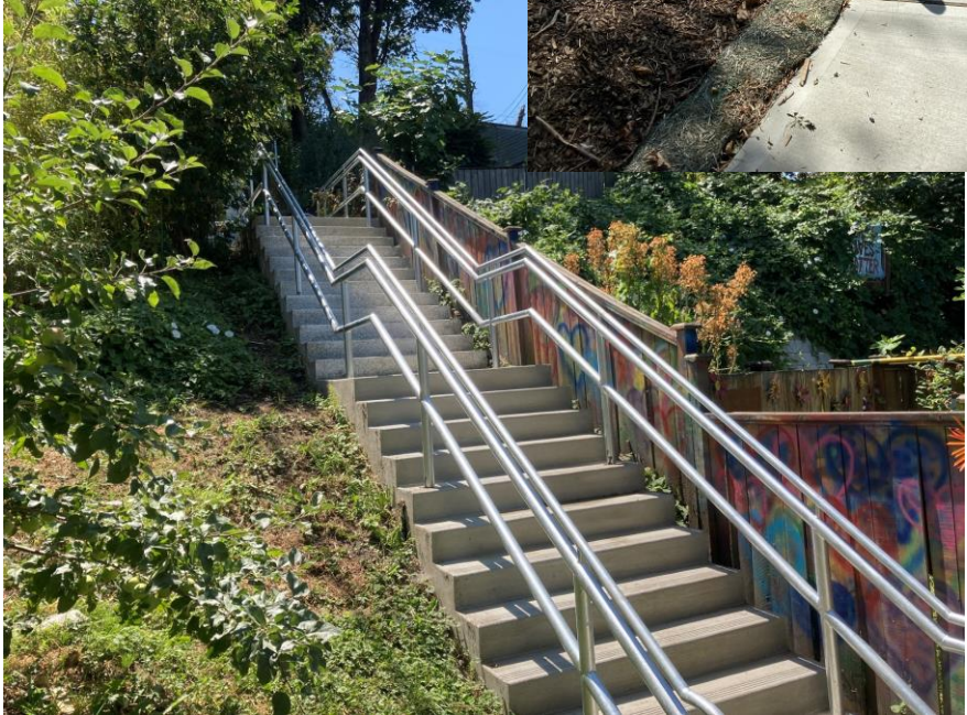
STW-353 10th Ave S & S Trenton St
