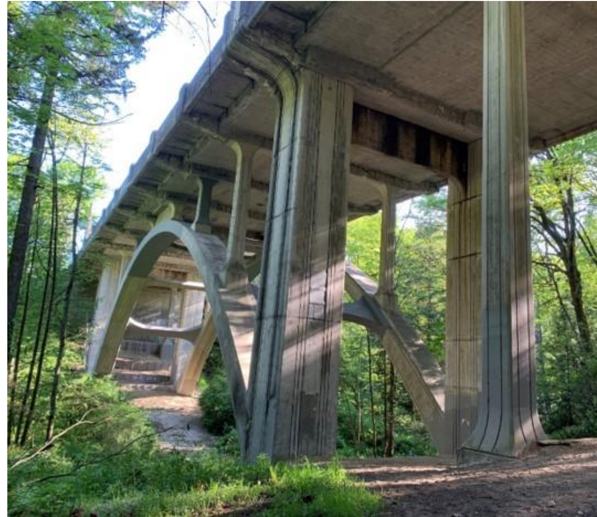
Underside of the Cowen Park Bridge showing installation of the carbon fiber wrapping on the arch support struts
