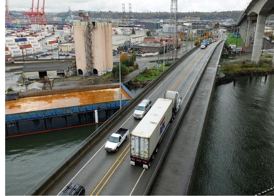
Lower Spokane Street Bridge
